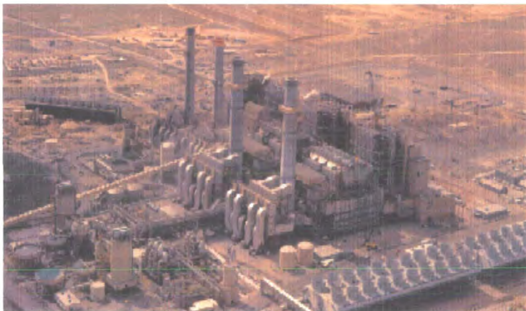
Illustration 1 World's largest regenerable FGD unit
