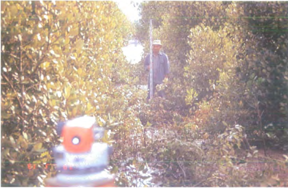
Fig. 5.16 Levelling and sampling across mangrove swamp, south bank of Kuantan river estuary. Note the straight line cut through the mangrove vegetation.
