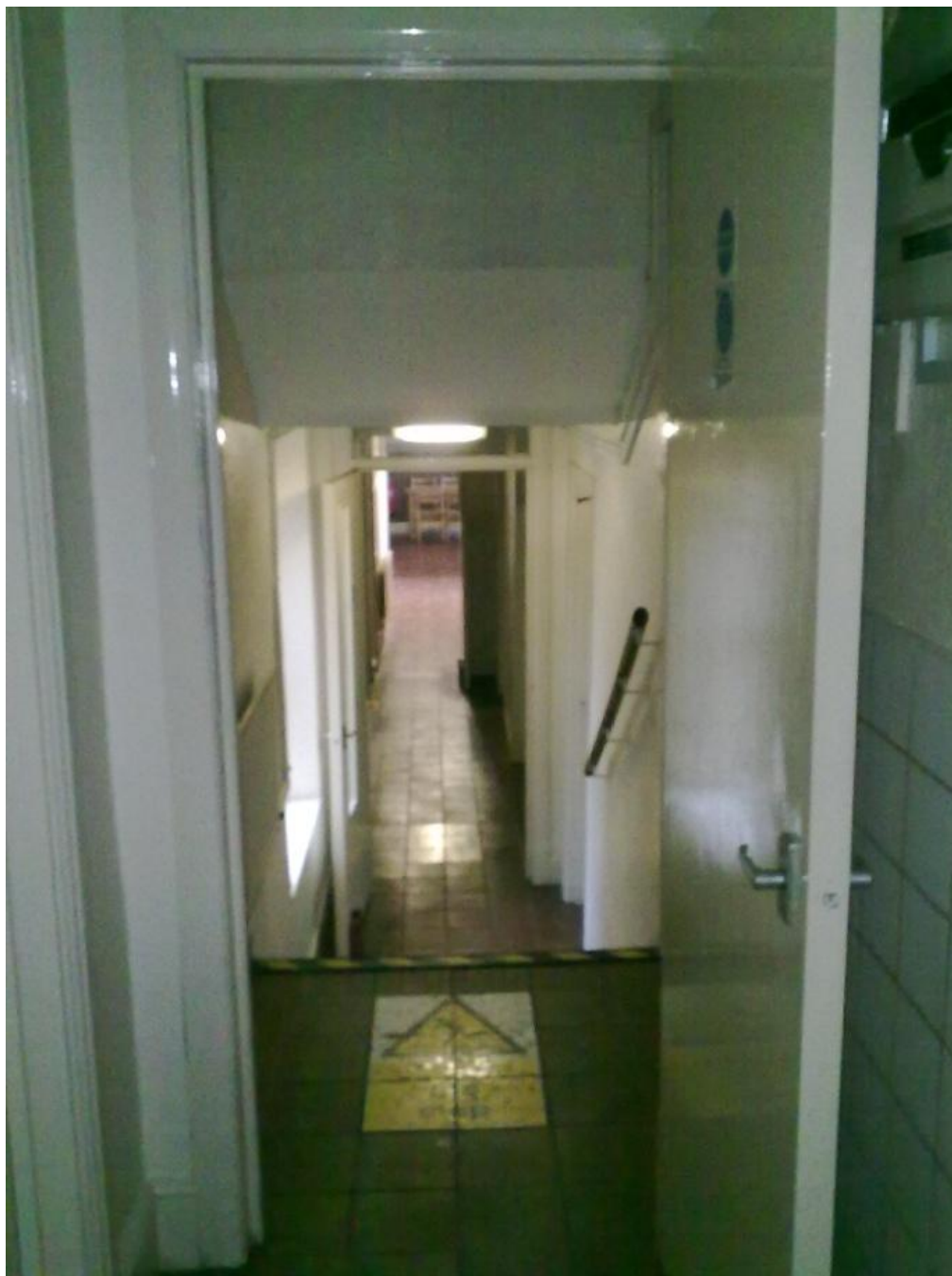
Figure 3 TH Ground floor hallway (to dining room)
