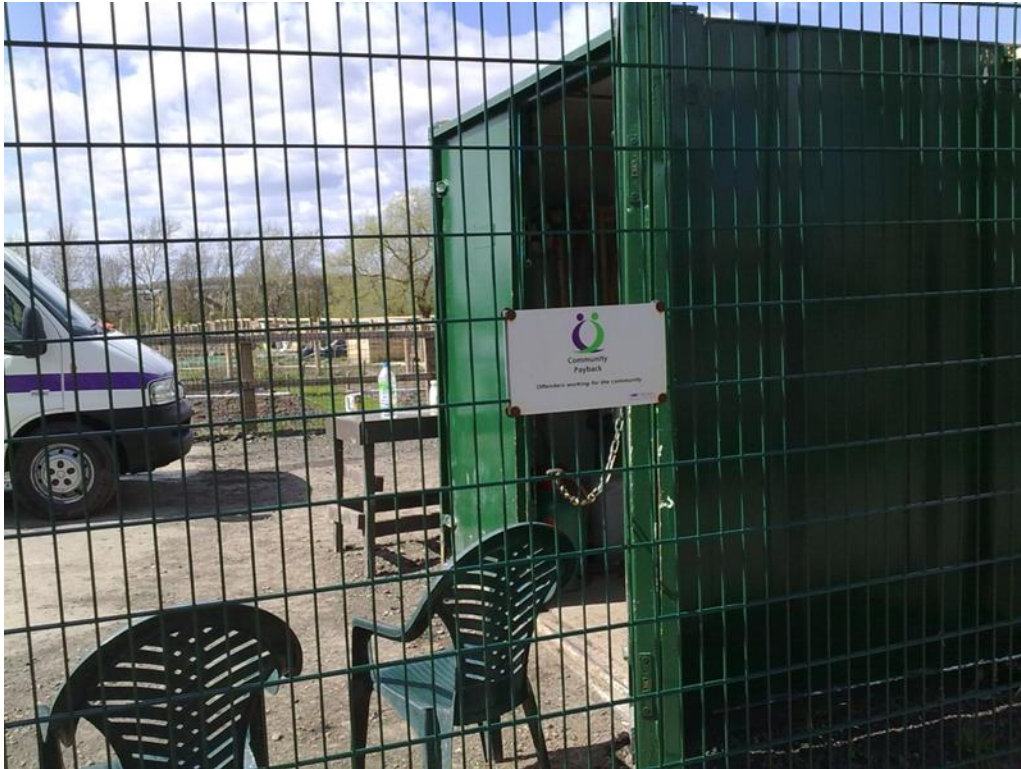
Figure 13: View of worksite from pavement
