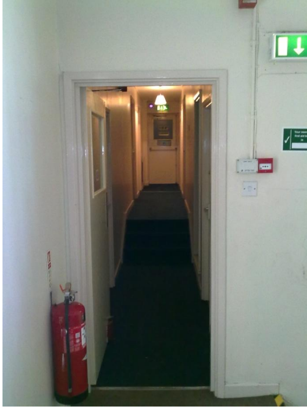
Figure 4 TH 1st floor hallway (to bedrooms)
