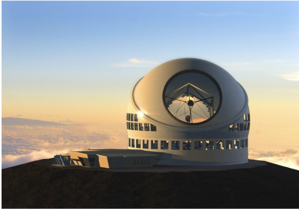
Figure 2.3: Rendered image of the TMT enclosure both the E-ELT and the TMT dome have chosen a round dome to minimize the turbulence at the surface and ground layer, hence reducing the wind loading. The enclosure is type "Calotte". http://www.tmt.org/observatory/enclosure-infrastructure . Credit TMT Consortium.
