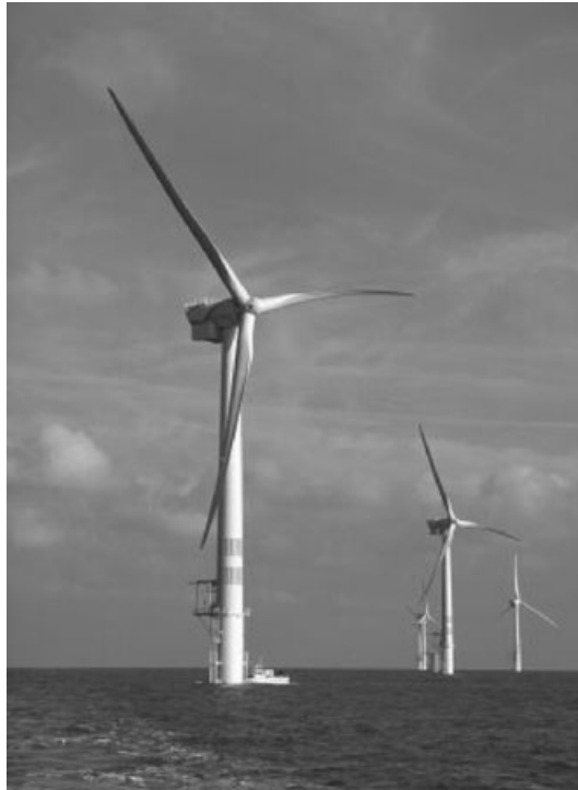
Figure 1. Typical Danish concept wind turbines as considered in this article (courtesy of GE Wind Power)
