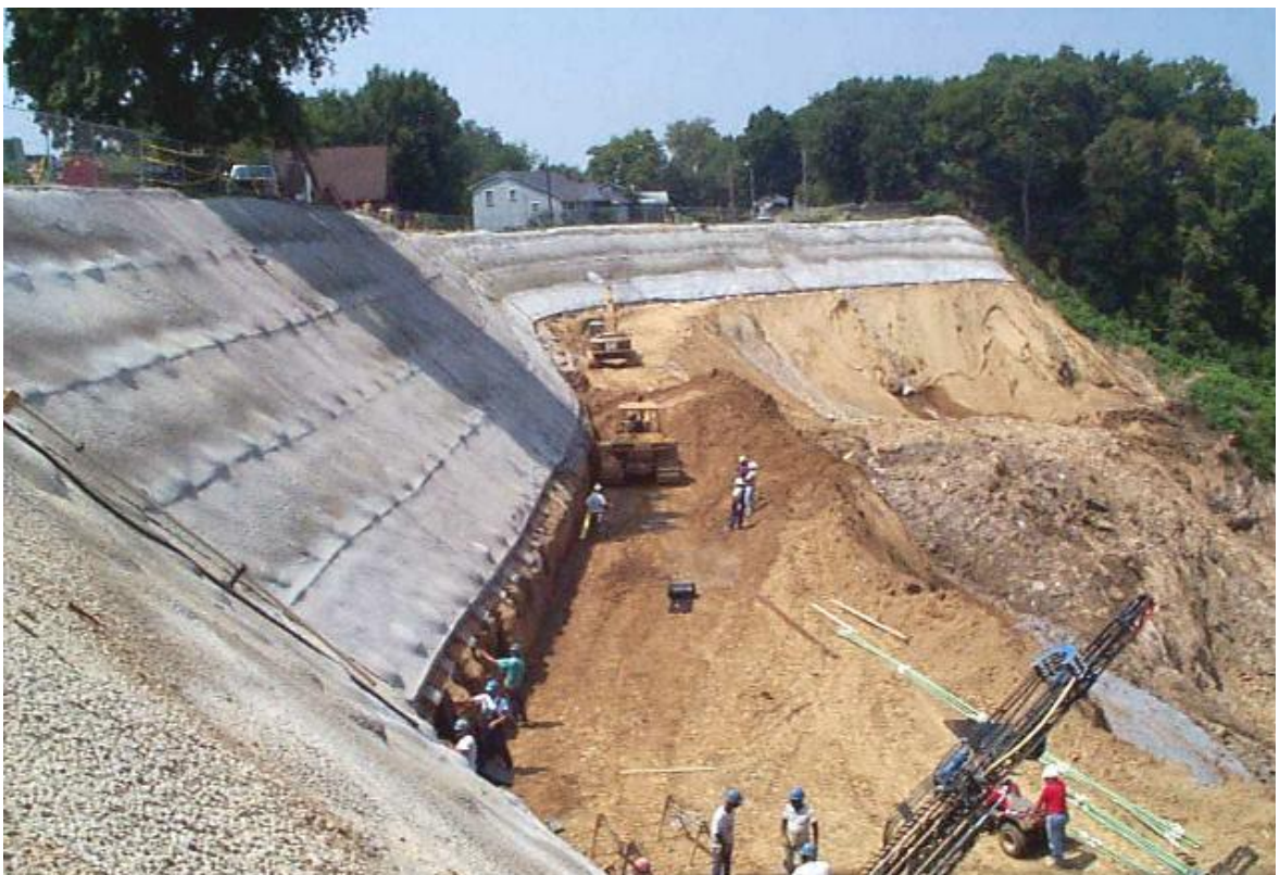
Figure 6.1: An example showing the use of steel rods and concrete to stabilise a hillslope.
