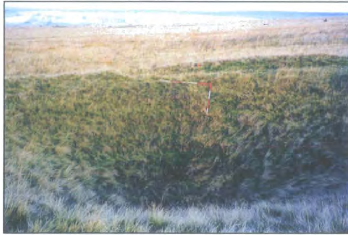
Figure 5.36: Baildon shaft of pronounced topographic expression (radius 8m)
