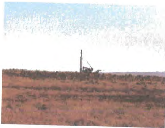
Pumping in the basalt.
