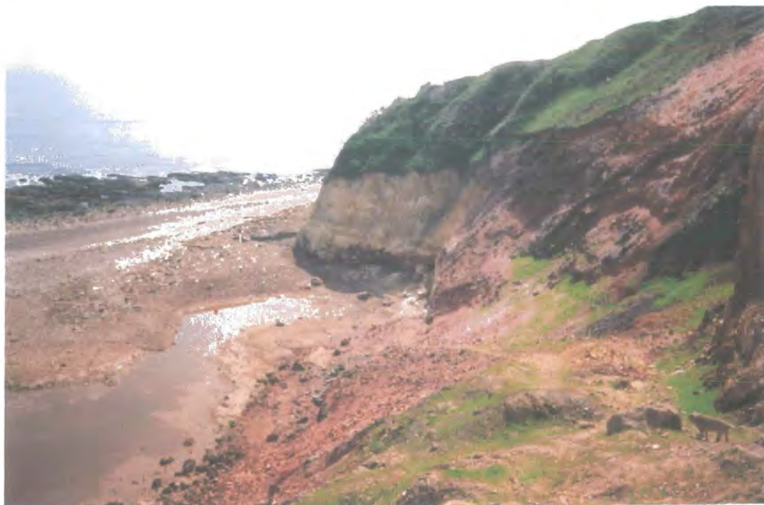
Plate 9.11 Easington Beach and Cliffs after TTT works
