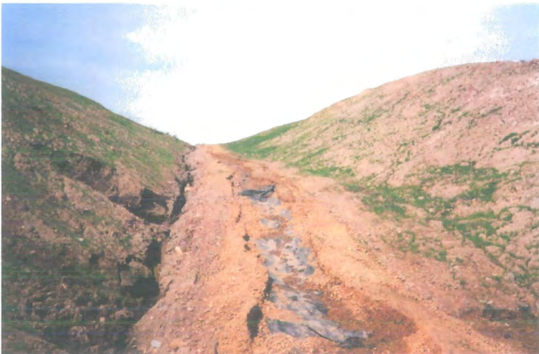
Plate 9.4 Work in Progress at Easington Colliery Beach May 2000
