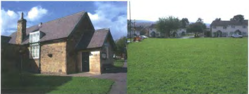
Fig. 44 The institute in 2006 and a view of the type of 1960s houses which replaced those demolished buildings shown on the photograph above (copyright author).
