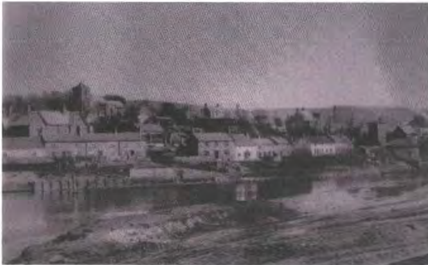
Fig. 25 Newburn in 1899 from the south bank of the River Tyne (copyright NCL, after Walton 1990). Of these buildings along the river frontage, which included old cottages called Water Row only the Boathouse Inn survives today. Water Row, was cleared by Newburn UDC as part of a 'slum clearance' in 1931-39 (TWAS UD/Nb/40/35). George Stephenson worked at Water Row Pit from 1798 to 1801.
