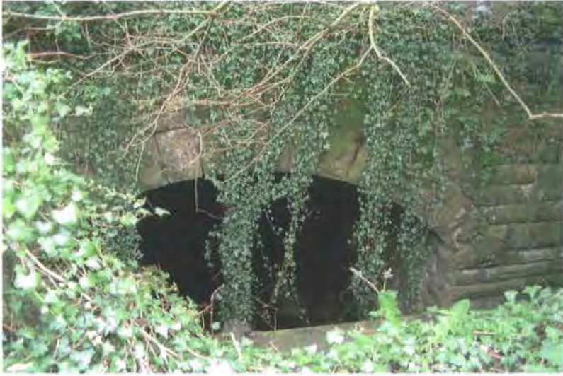
Fig. 149 Eighteenth century skew bridge, which carried the Wylam Waggonway over the New Burn, Locally Listed (copyright author).
