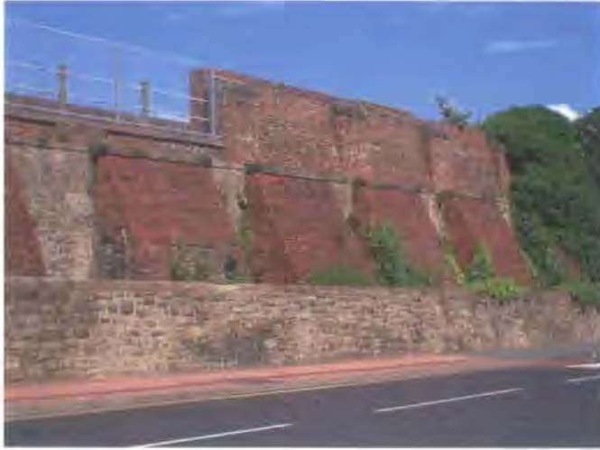
Fig. 107 Substantial brick and stone retaining walls still hold up the Throckley Filter Beds high above Hexham Road. They are a prominent architectural feature (copyright author).
