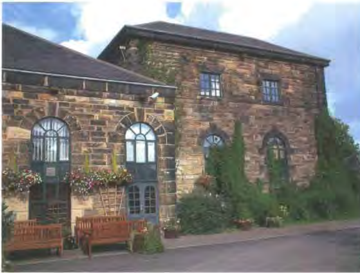
Fig. 105 Newburn Water Pumping Station constructed by R. Cail in 1855 for the Whittle Dean Water Company, now the Keelman Public House, listed grade 2 (7/29). (copyright author)
