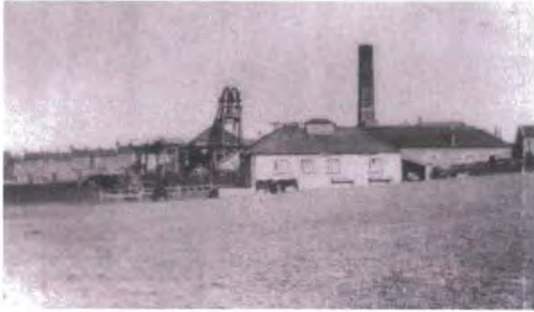
Fig. 84 Blucher Colliery whilst in operation by Throckley Coal Company between 1901 and 1924 (after Peacock 1994). The photograph shows an extensive range of colliery buildings, a chimney, the headstock and the miner's cottages to the rear. Next to the colliery the fields remain as grazing land, showing that mining and agriculture co-existed.
