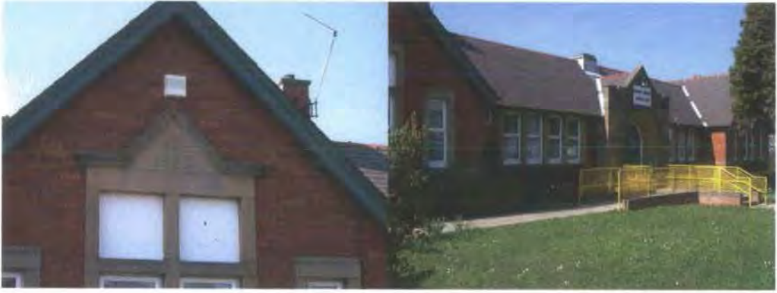
Fig. 59 This institute, dated 1925, was built next to the in-filled whinstone quarry, along with a recreation ground and football pit (copyright author).
