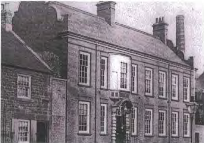
Fig. 121 Spencer's offices, Newburn High Street – in the background is one of the steelworks chimneys. The shaped gables echo the design of the Duke's almshouses (see chapter eight). (copyright Newburn Library).
