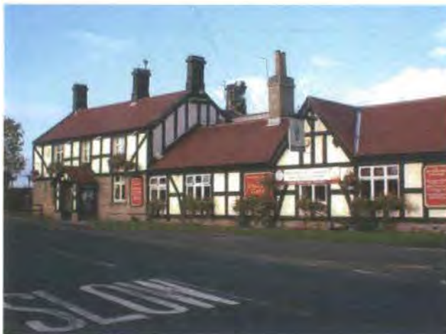
Fig. 146 Jingling Gate Public House, Stamfordham Road (copyright author). Located on a major routeway into Newcastle, the public house would have provided welcome refreshment for travellers and stabling and blacksmith's facilities for their horses.
