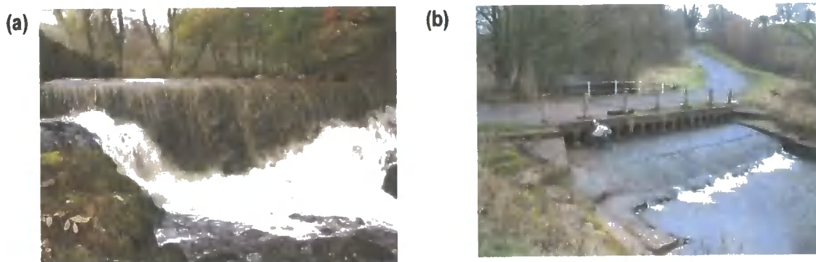
Figure 3.13: Impassable barriers to salmonid migration found in the Eden catchment, (a) Swindale Beck Upper Weir and Cam Beck Pipe Bridge. Photographs courtesy of Eden Rivers Trust.
