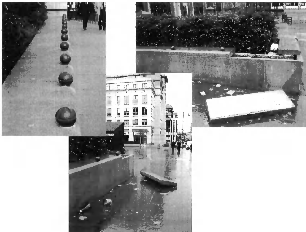
Figure III.5: Displaced slab on the SE corner of Festival Square.
