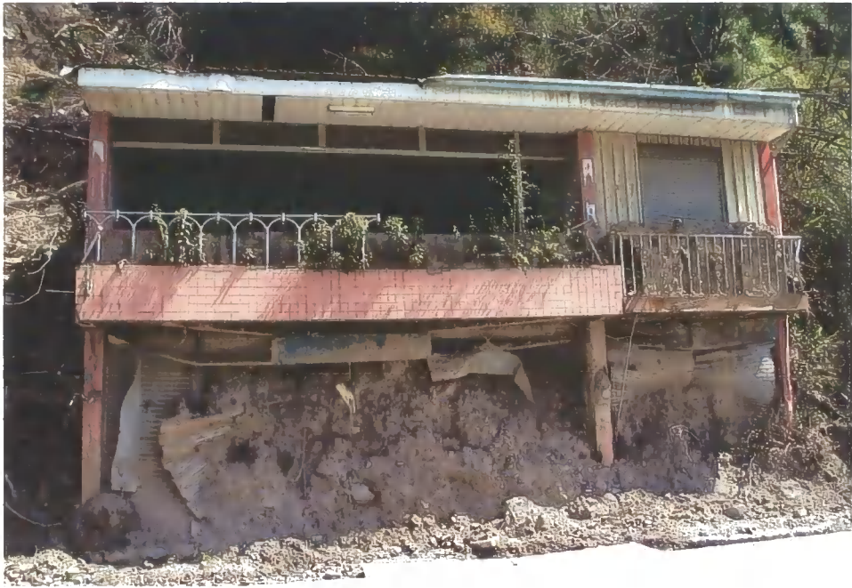
Figure 3.1 A fatal landslide event along the Route 21 highway, near Shenmu, Chenyulan Stream area, Central Taiwan.
