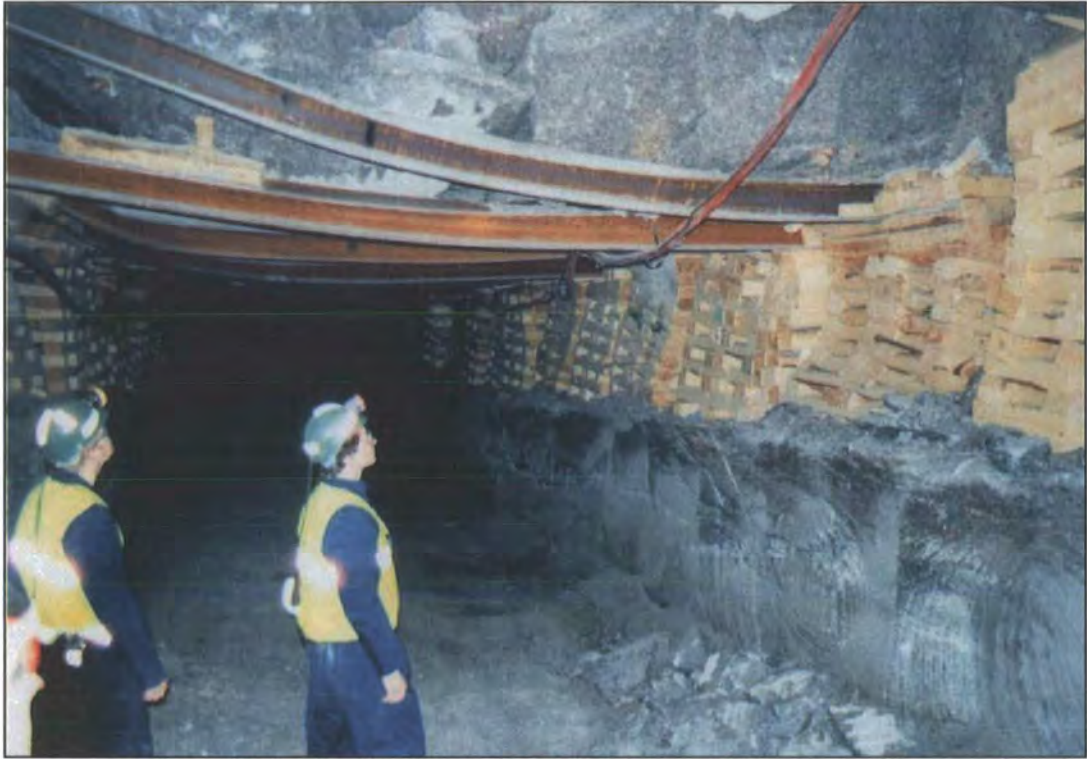
Figure 3.20: Boulby mine - limited closure in salt workings, kept open for transport.
