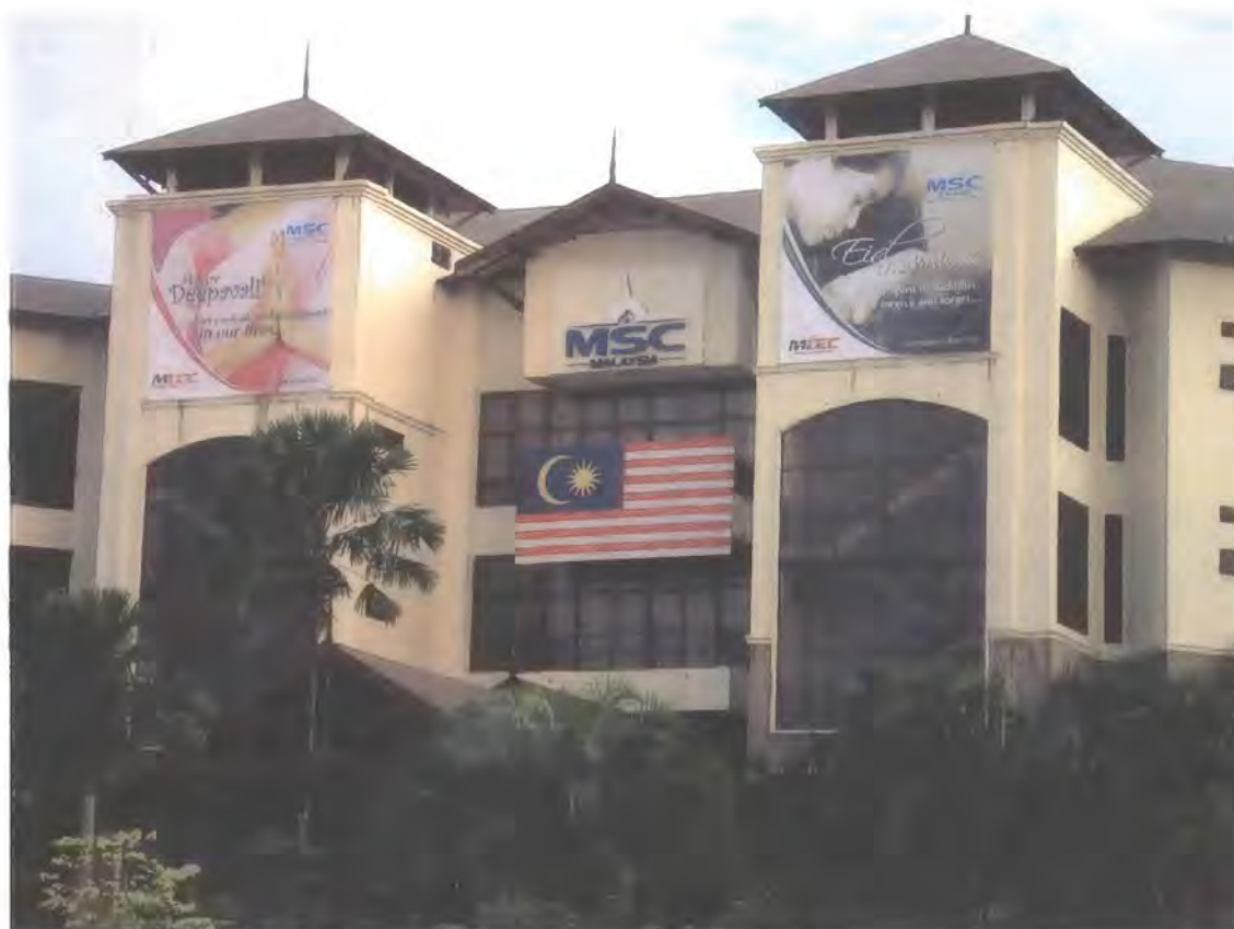
Figure 22: Multimedia Development Corporation HQ, Cyberjaya (Source: Author's Photograph)
