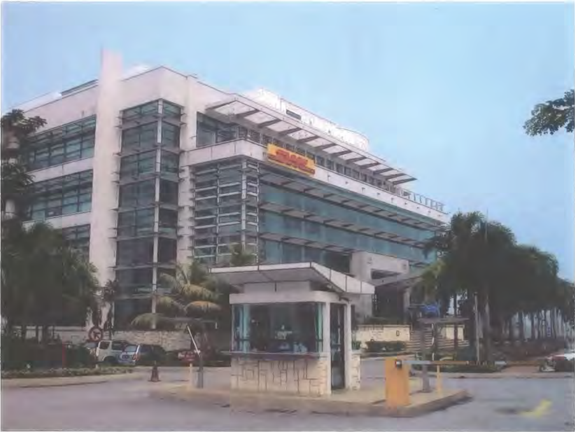
Figure 28: DHL Global Data Centre in Cyberjaya (Source: Author's Photograph)
