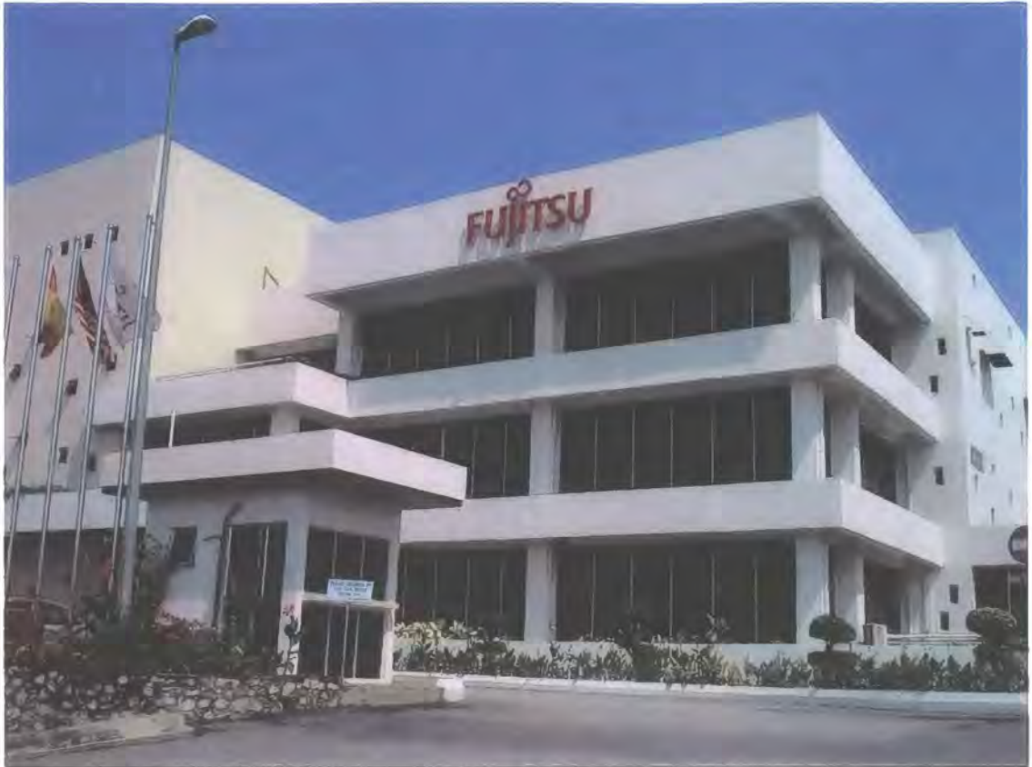
Figure 19: Fujitsu Office in Cyberjaya Exemplifying the 'International Style' (Source: Author's Photograph)
