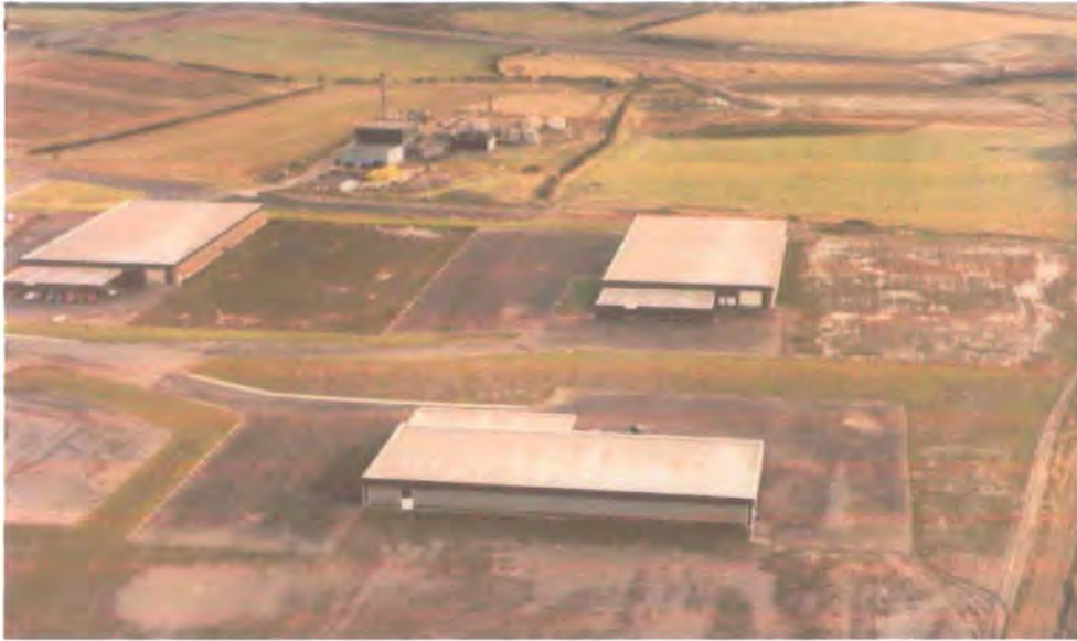
Fig. 20: Advance factories being erected to the west of the A19 at Peterlee.
