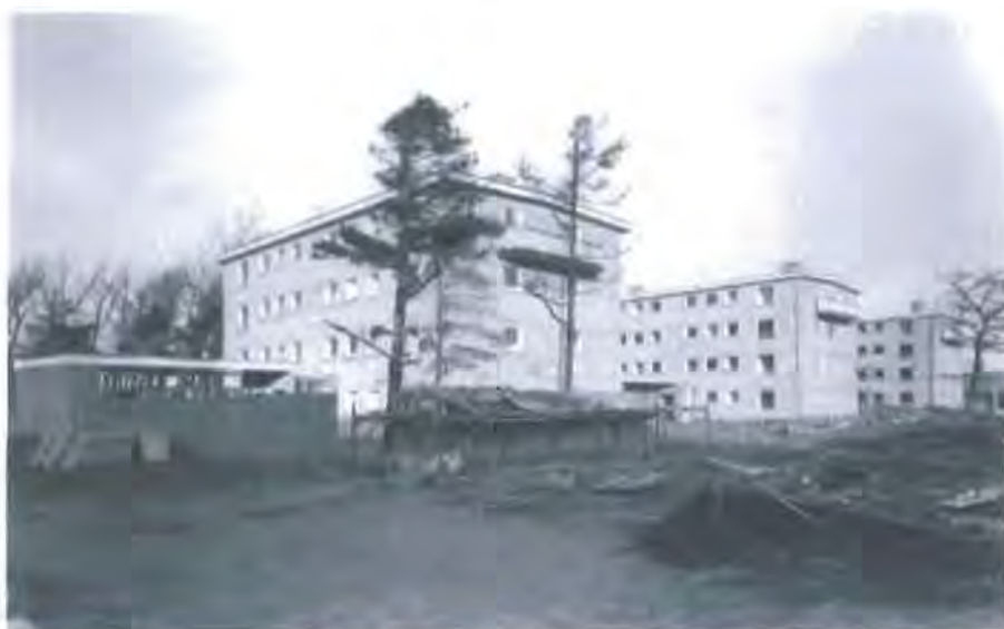
Fig. 6: Flats constructed in Aycliffe by the corporation's direct labour dept.
