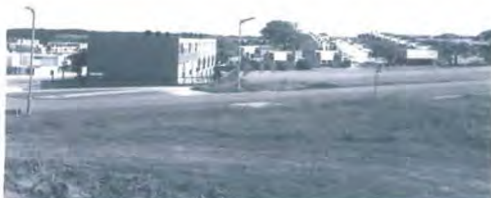
Fig. 11: Pasmore-designed flat-roofed houses in the south-west area of Peterlee.
