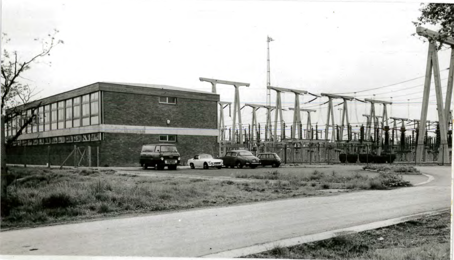
Photograph 51. Control building at South Manchester substation. Nearly every primary grid substation has a control building similar to the one shown in this photograph, usually two storey, but occasionally single storey. It is manned continuously for the operation of the transformer and switches, as well as providing for the security and supervision of the substation. The main room is the control room which occupies most of the first floor. The ground floor provides accommodation for banks of relay panels, and the electronic apparatus required for telecommunication with national control in London, and a local area control in Manchester.
