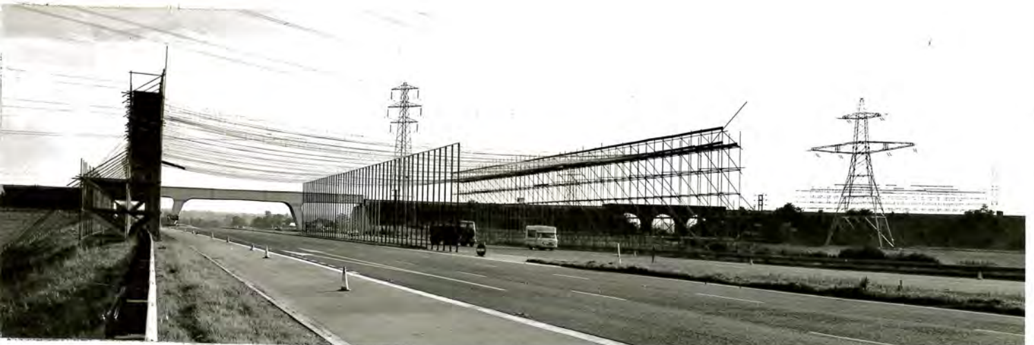
Photograph 6. Showing the extensive scaffolding required to support conductors during construction across the M.4 motorway.
