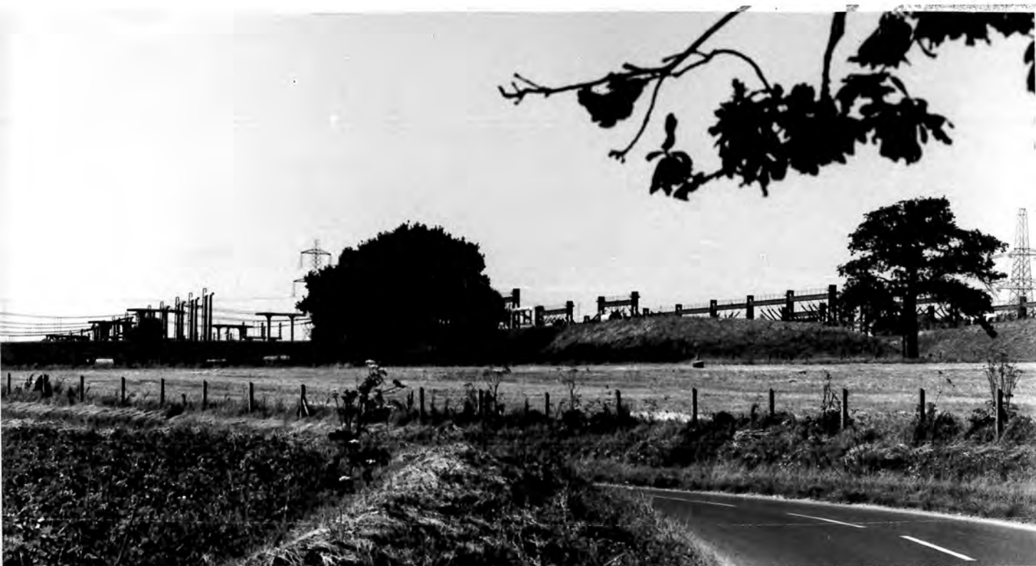
Photograph 78. Lovdean substation, taken in October 1966, soon after the completion of the ground modelling.
