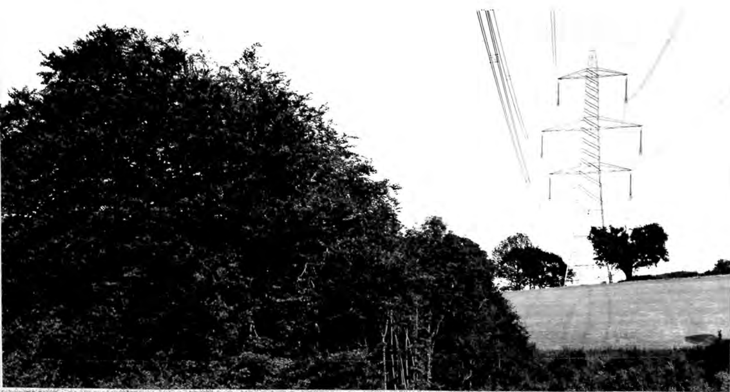
Photograph 15. A section of the Lydd-Bolney 400 kV line near Hurstmonceaux, Sussex. The two trees under the line were cut at the owners insistence to the minimum required to meet the electrical clearance regulations, and no reshaping of these trees was done. The tree in the foreground is a large Copper Beech, and this was lopped and side pruned by about 20 ft., and reshaped to conform to the natural shape of the tree.
