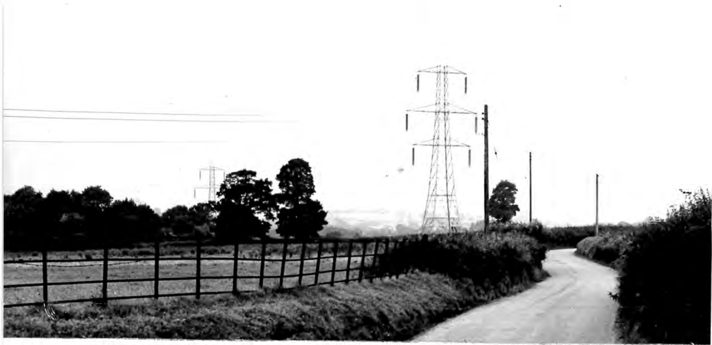
Photograph 67. 275 kV straight line tower conspicuously sited alongside highway.
