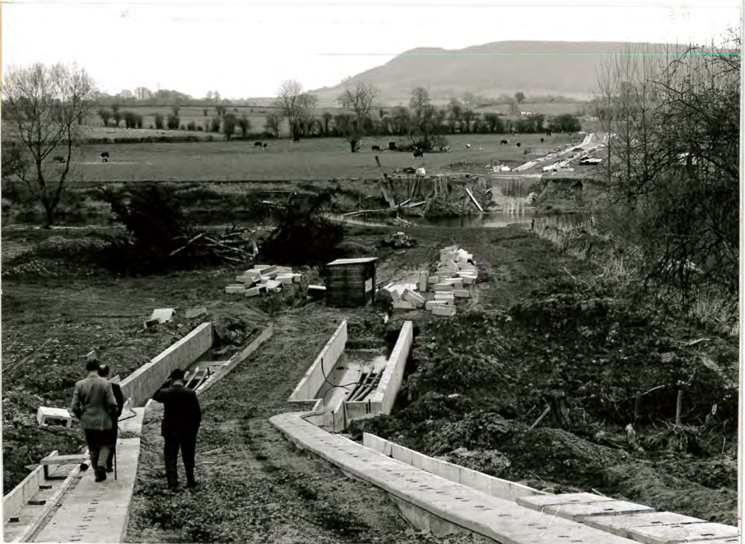
Photograph 35. Installation of concrete troughs for 400 kV cables at approach to the River Wye.
