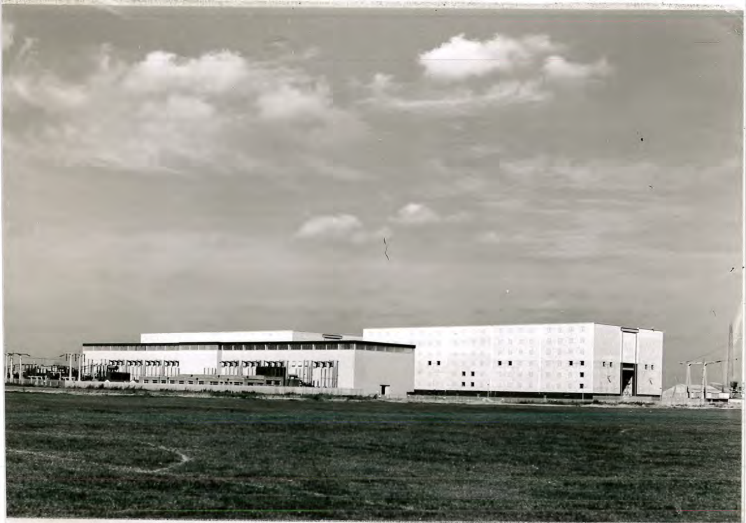
Photograph 47 showing 132 kV switchhouse in foreground and a 275 kV switch-house behind at Willesden. The Board justifies the cost of these buildings on the ground that this was the only way to get all the electrical equipment required on to this restricted site.
