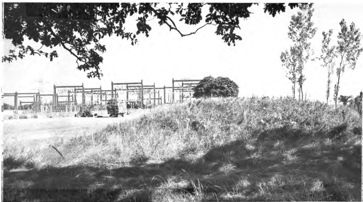
Photograph 36 of a 400 kV substation showing the 70 ft. high steel gantries required for supporting live electrical equipment, described by the Board as the Mark I design. All the Board's 400 kV substations have been built so far to this design.
