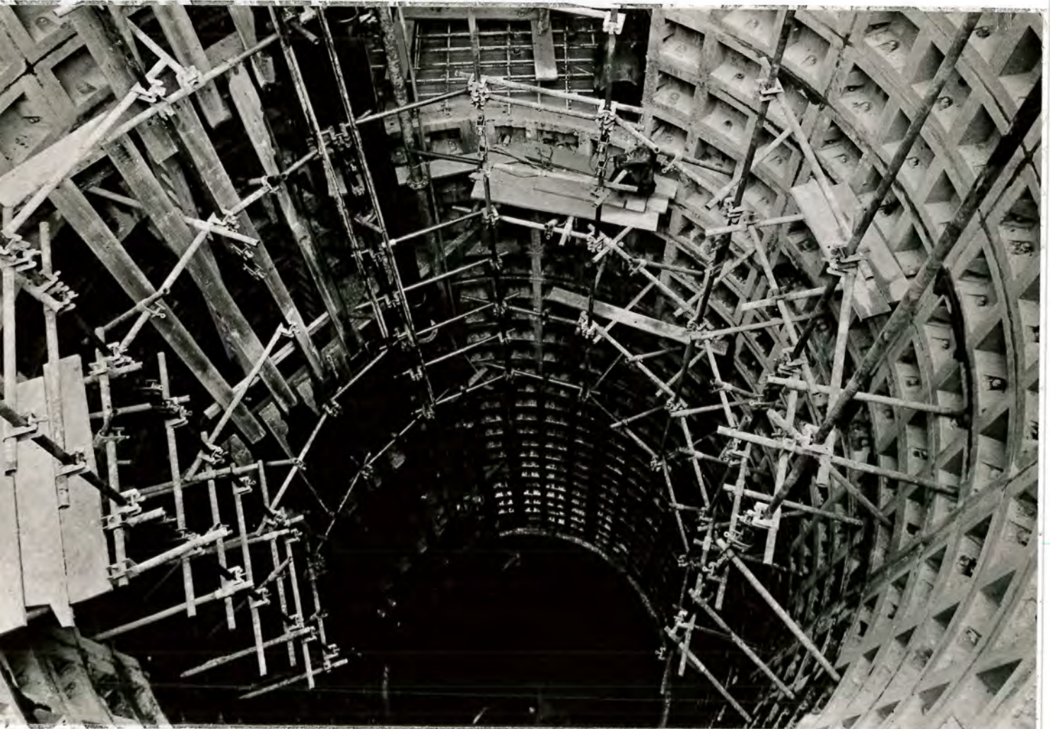
Photograph 34. Vertical cable shaft at Tilbury under construction.
