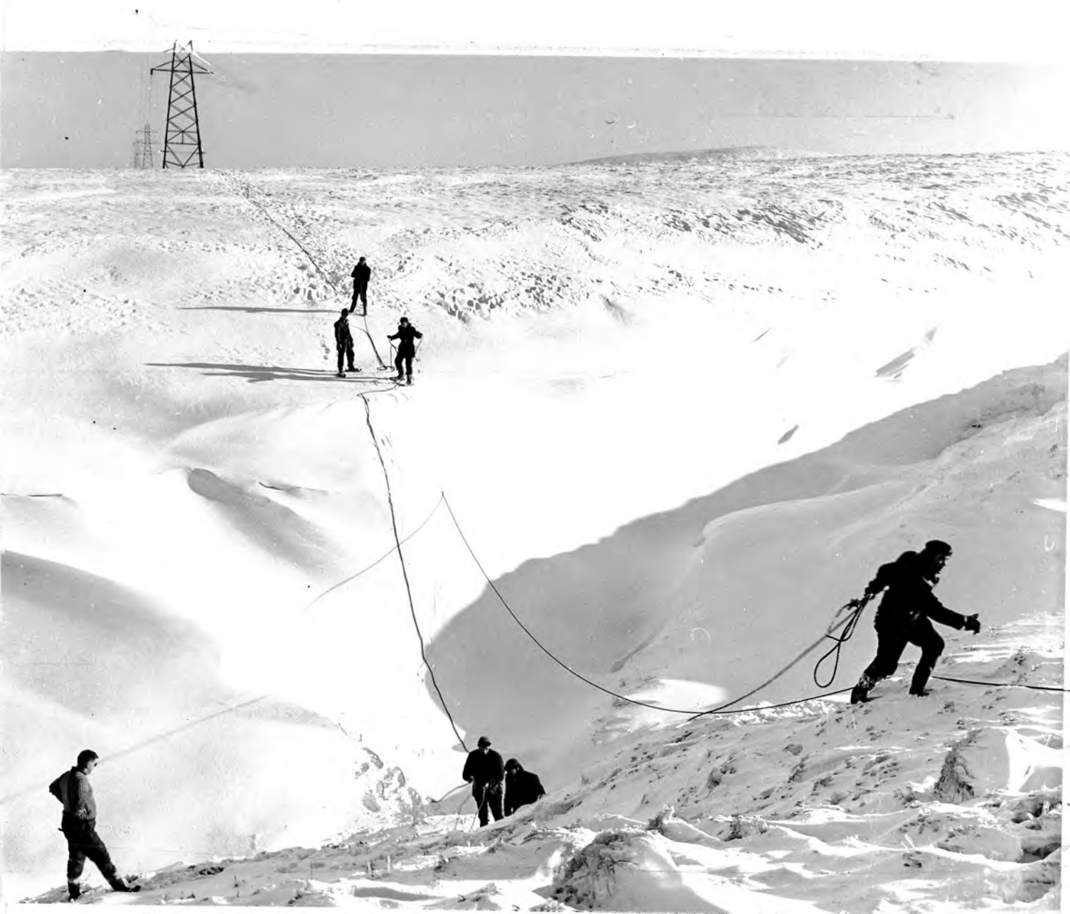
Photograph 3. Broken conductors on a 132 kV line in South Wales caused by snow and high winds during the winter of 1963. The difficulty of repairing lines under these conditions suggests that lower and more sheltered routes for transmission lines should be chosen if possible.
