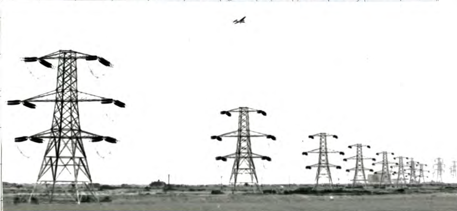
PHOTOGRAPH 8 REDUCED HEIGHT TOWERS CLOSE TOGETHER WITH TENSION INSULATORS. NOTE STANDARD HEIGHT TOWERS TO RIGHT OF PHOTOGRAPH
