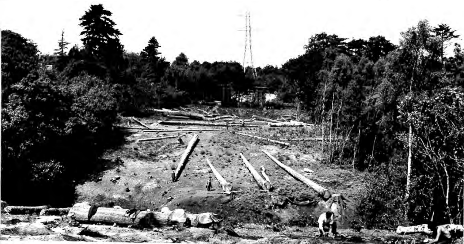
Photograph 17. A section of the Ninfield-Hastings 275 kV line under construction adjoining Claremont School near Hastings, showing deliberate uneven felling along the sides of the swathe to give a more natural effect. The scaffolding near the tower is to carry the conductors during erection to avoid damaging or felling the trees near the base of the tower.
