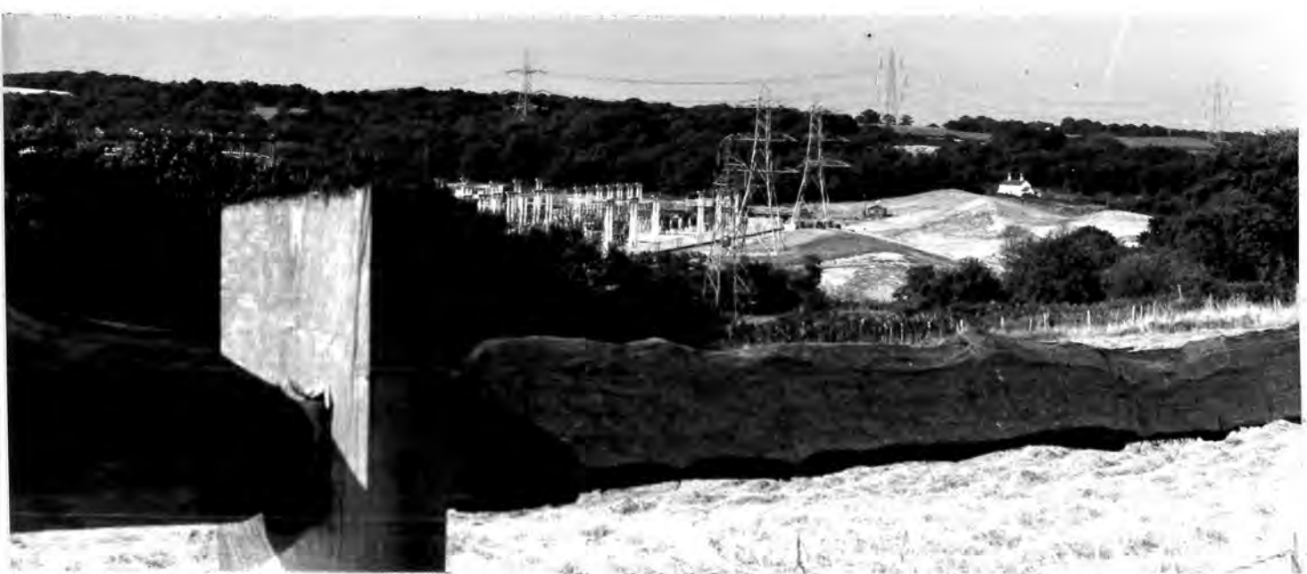
Photograph 40. Ninfield substation is regarded by the Board as one of the best examples of good siting from an amenity point of view. The substation structures that were coloured grey are barely distinguishable in the top left of the photograph.
