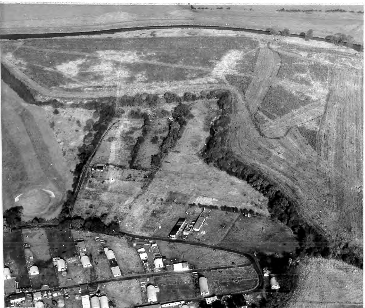
Photograph 50 showing site of South Manchester substation before construction, and the piggery smallholdings the retention of which required an expensive modification to the substation layout.
