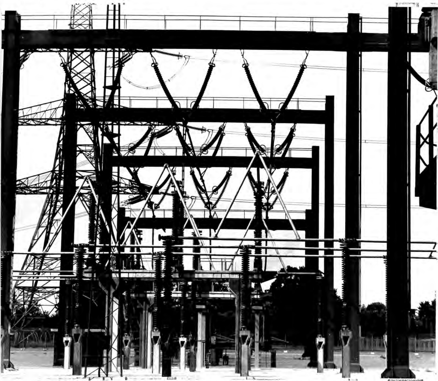
Photograph 38. Interior view of Enderby 400 kV substation showing 70 ft. high steel gantries, and the aluminium bus bars carried on stacks of insulators mounted on concrete posts. The 8 ft. high security fence helps to give some impression of the large size of this electrical equipment.
