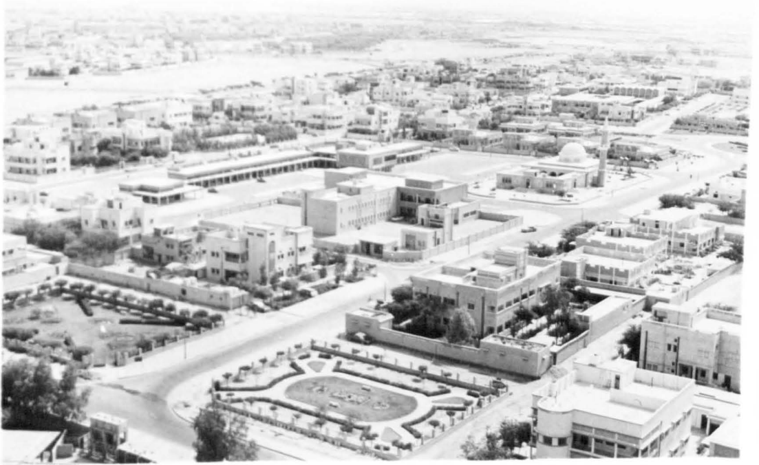
Plate 11.1 Shuwaikh Co-operative Centre. Note the rectangular layout of the roads.
