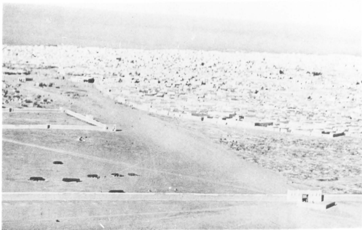
Plate 7.1 Mirqab in the 1930s. Note the space between the edge of the town and the wall.
