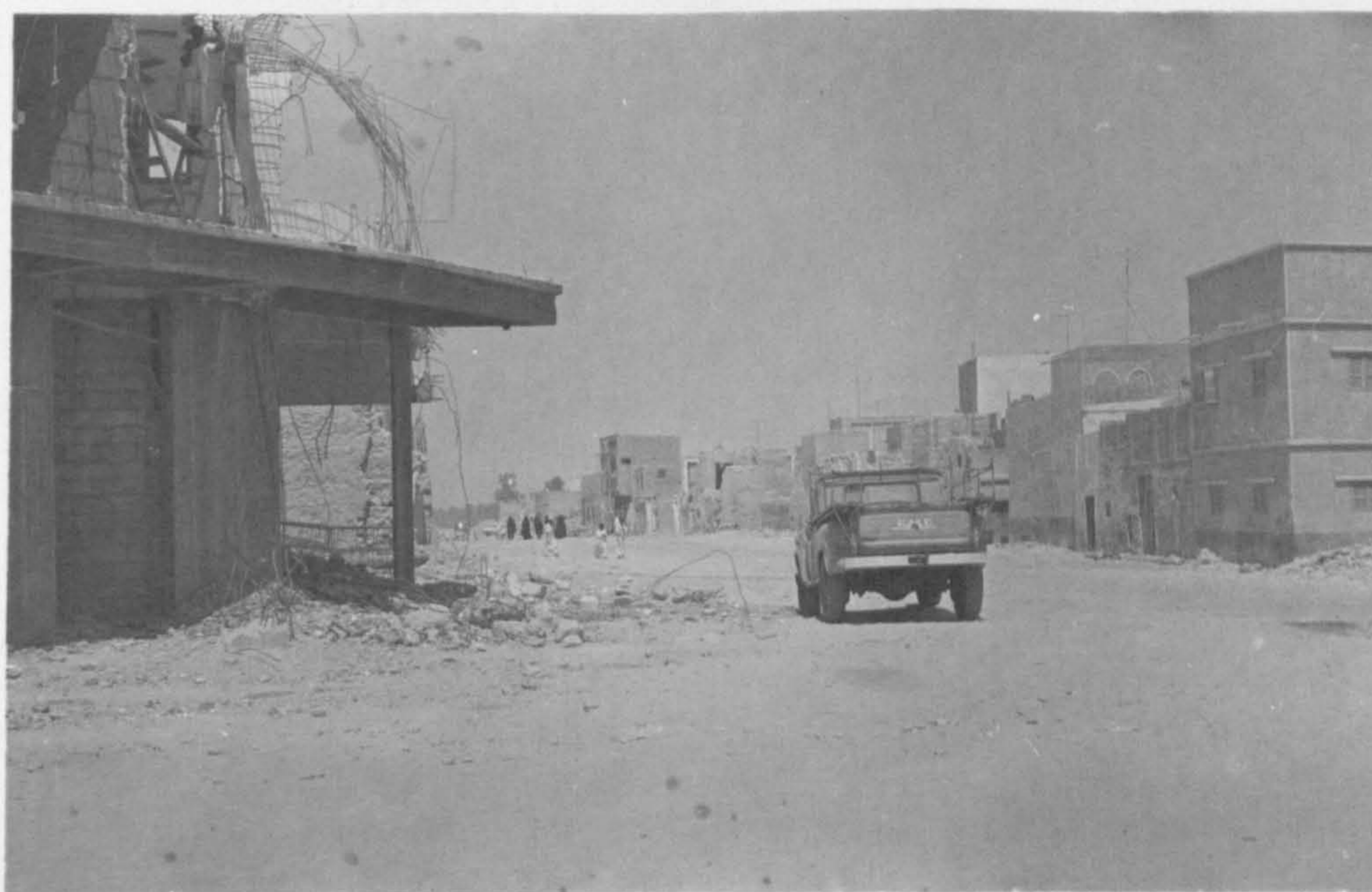
Plate 13.11 The size and position of first-floor windows depends largely on the distance between them and the house opposite, and the expected future development of the area opposite, as well as on the attitude of the occupier
