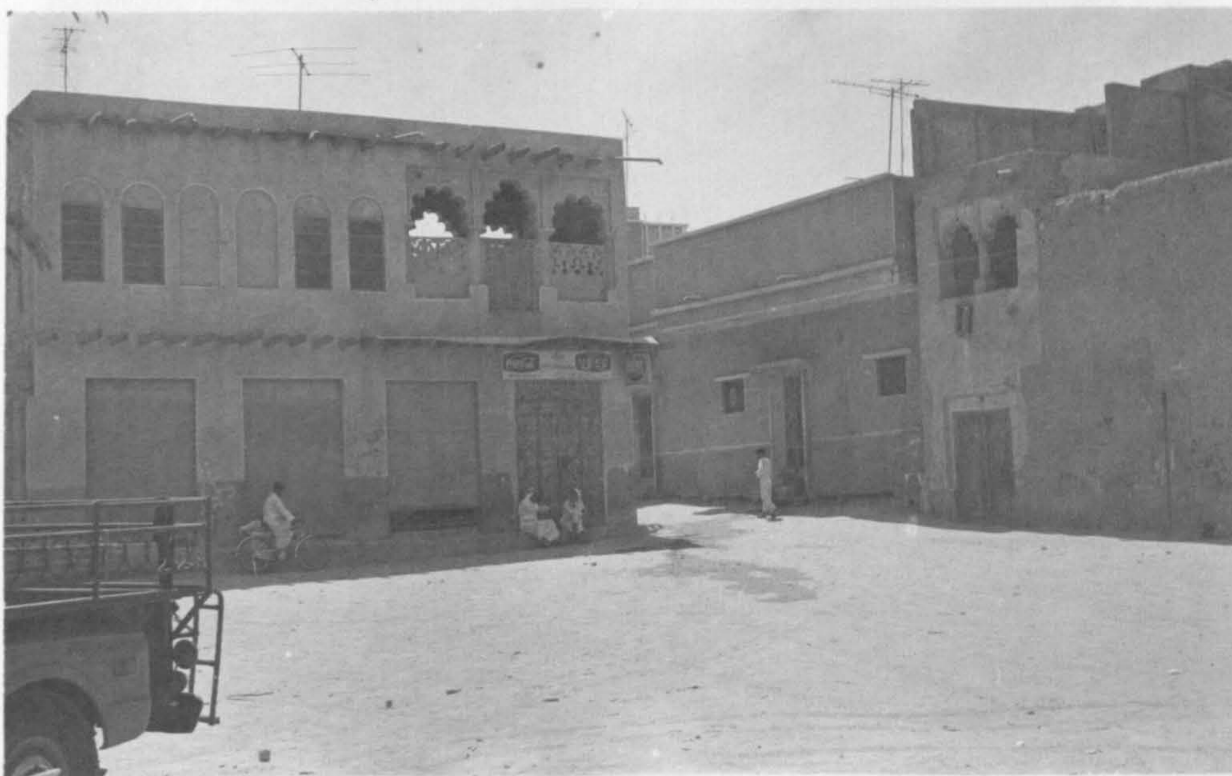
Plate 13.10 Windows in the grand floor are small and placed high in the wall for protection against the intruding eyes of the passer-by
