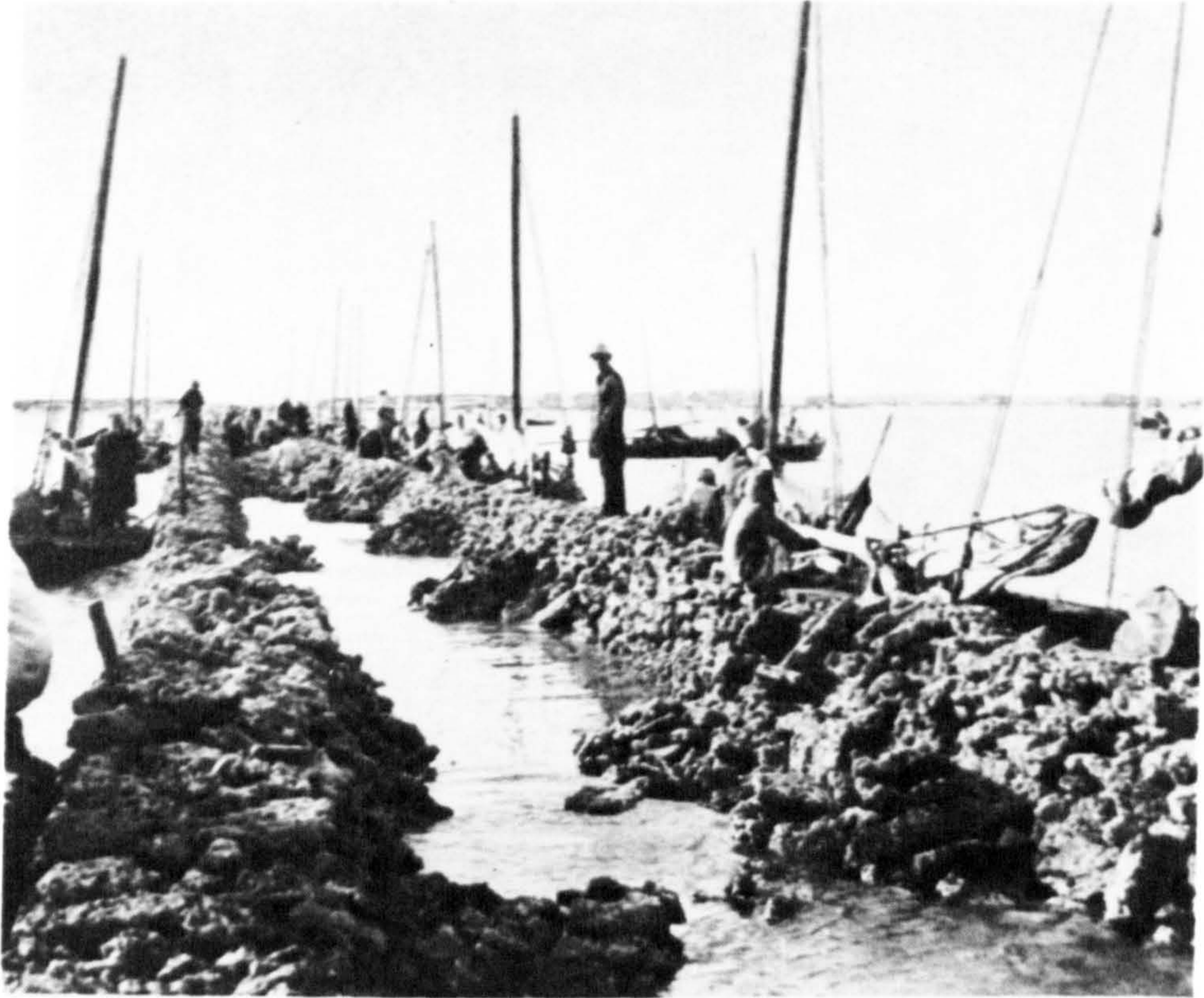
Plate 4.1 The building of Al-Khobar pier in 1934-35 afforded the first construction jobs provided for local people by Aramco Oil Company
