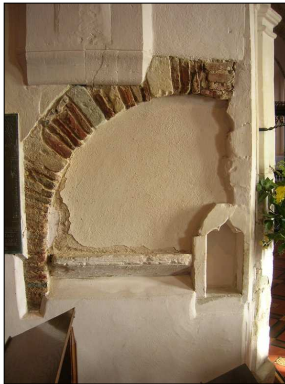
Fig. 3.72: Small niche in the wall north of the opening between the nave and tower. The pattern of construction (brick and stone voussoirs) is the same as the original chancel arch (see Fig. 3.71).
