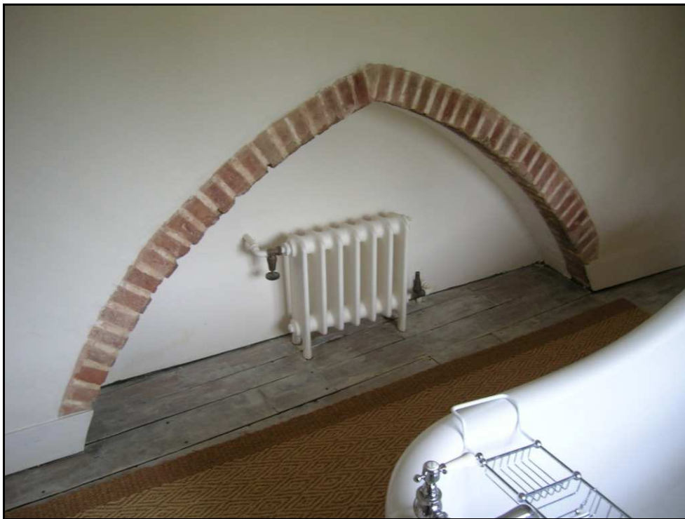
Fig. 3.8: The top image shows the Infirmary column with scalloped capital, now highly worn. The springing for the lancet arch can be seen above the capital whilst the crown of the arch is seen in the bottom image.
