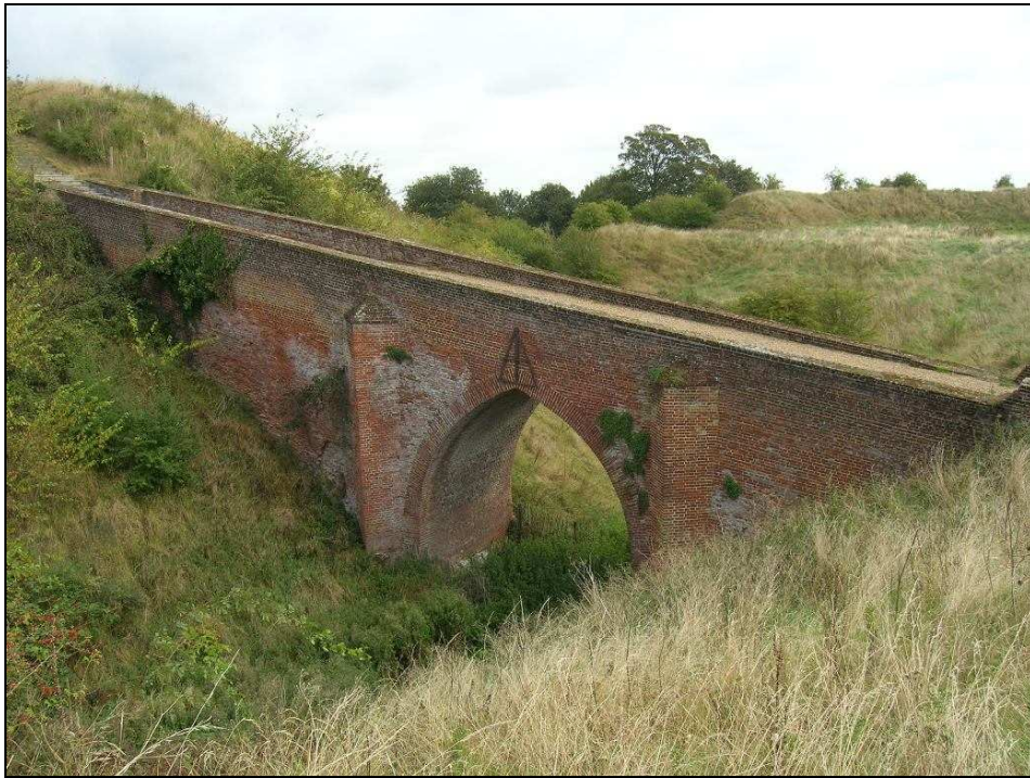
Fig. 2.15: Brick bridge at Pleshey Castle connecting the motte and inner bailey.
