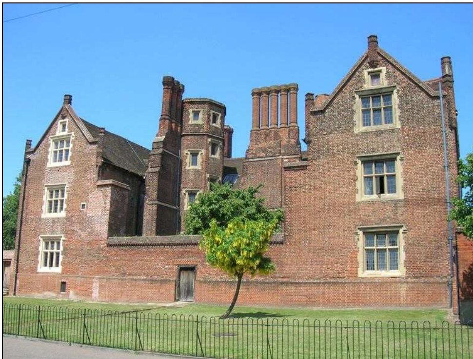
Fig. 3.15: Eastbury Manor House from the south.
