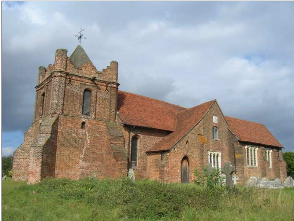
Fig. 3.84: All Saints' church, East Horndon. Note the combined southern transept and porch.
