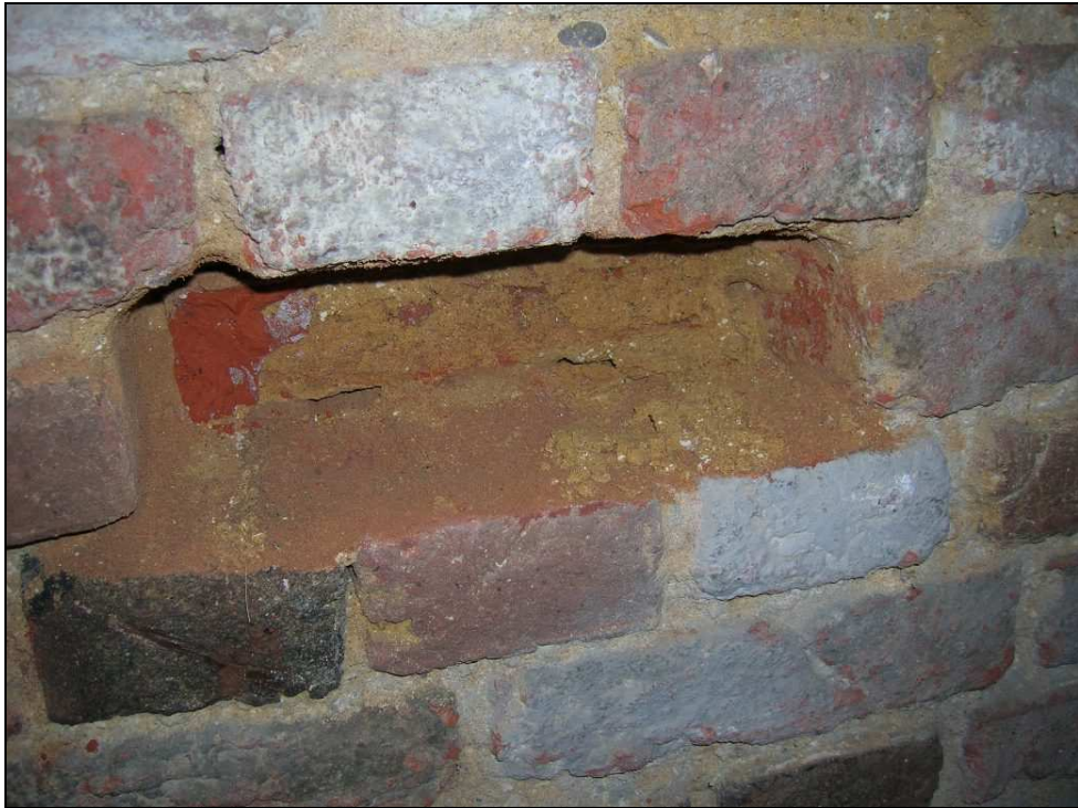
Fig. 3.106: The space where the sampled brick was located. The mortar surrounding the brick was drilled away before the entire brick was removed so that a sample could be taken from the rear surface to reduce the aesthetic impact.
