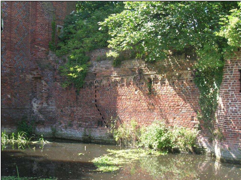
Fig. 3.46: The wall attached to the east side of the gatehouse. The dashed line represents the approximate location of the transition from high quality craftsmanship (to the left of the line) and poor quality craftsmanship (to the right of the line).
