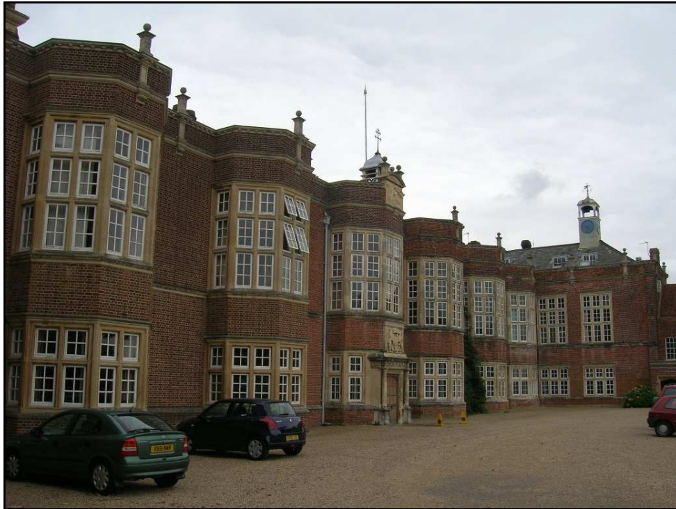
Fig. 3.49: Principle frontage to the late 16 th century building showing the bay window complexes. Note the main entrance into the centre of the range.
