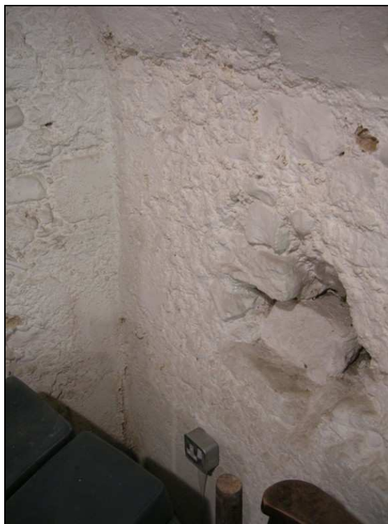
Fig. 3.95: Blocked indent at the eastern end of the southern wall of the sunken chamber. This feature might have been a piscina originally intended to serve an altar located at the east end of the chamber.
