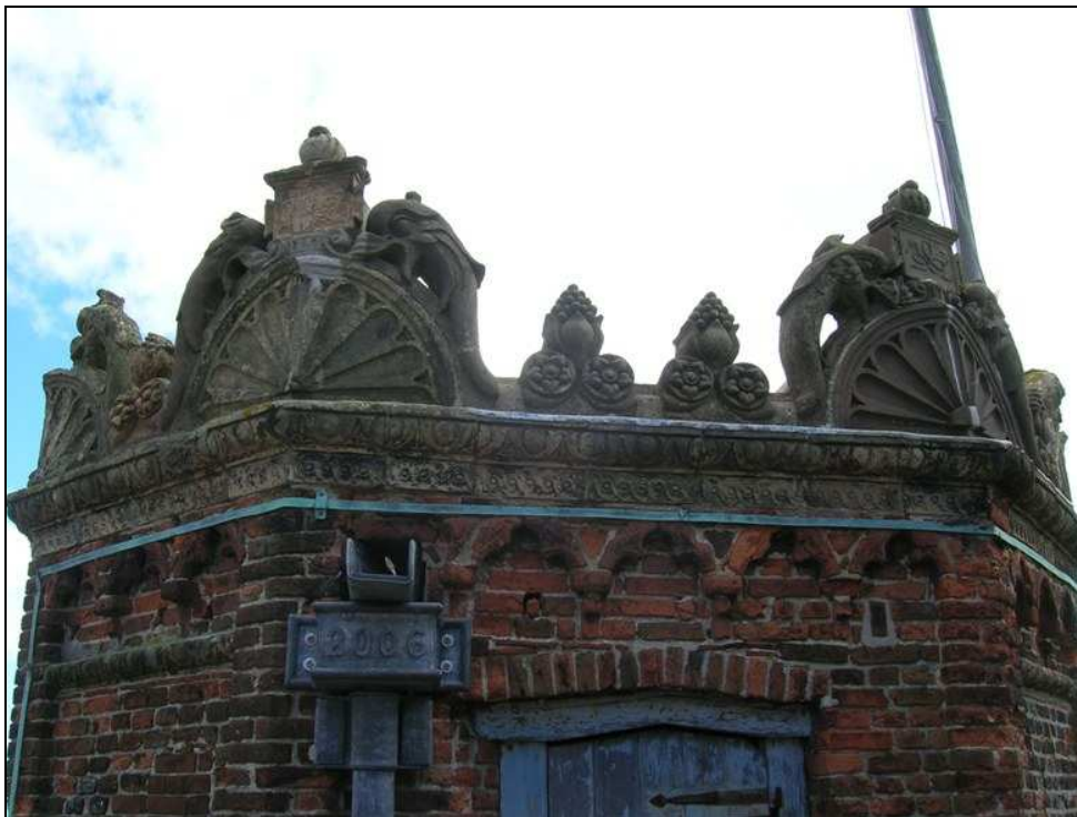
Fig. 3.27: Terracotta decoration on top of the gatehouse western tower.
