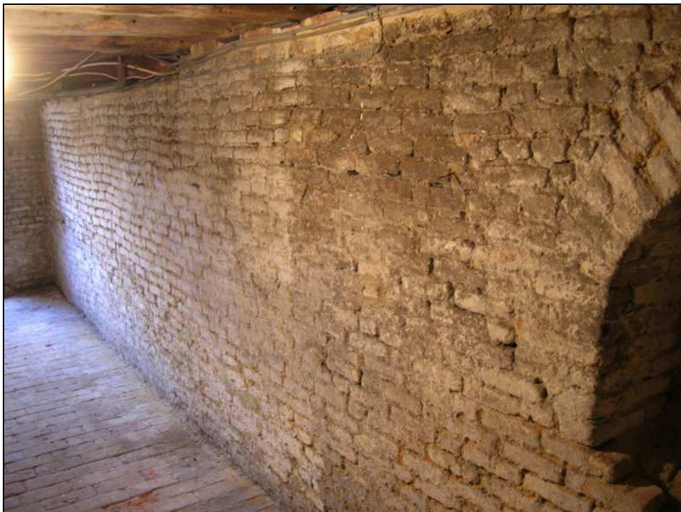
Fig. 3.62: The southern wall of the cellar, illustrating the extensive use of 'Flemish' type bricks.
