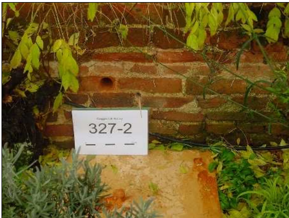
Fig. 3.13: The brickwork immediately around the sample location on the northern range at Coggeshall Abbey. Note that the two top courses of brick comprise the string course which connects the north range to the porch. The scale bar is 20 cm in length.
