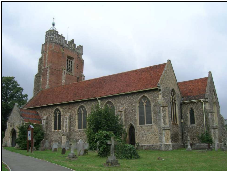
Fig. 3.79: St. Andrew's church, Earls Colne, seen from the south east. Note the extensive brick element on the eastern face of the western tower.
