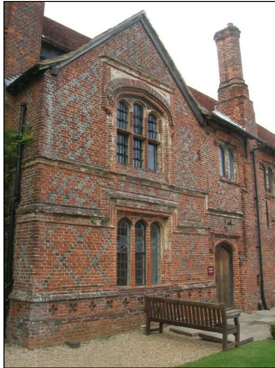
Fig. 3.25: The cross wing gable end at the western end of the eastern wing. Note the string course below the upper window which continues further around the building and the stone spandrels to the upper window.
