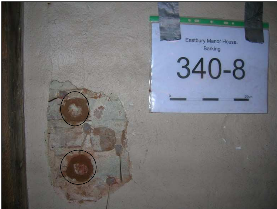
Fig. 3.22: The south western corner of the attic space where two samples were collected. The sample points have been circled. The scale bar is 20 cm in length. The image shows the wet mortar repair work shortly after sampling had taken place.
