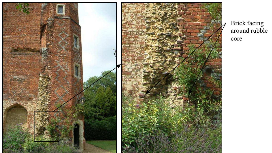
Fig. 2.18: Brick facing around rubble core on south eastern corner of the inner courtyard gatehouse at Leez Priory.
