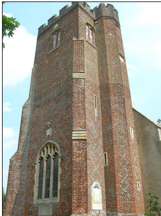
Fig. 3.108: The western brick tower of St. Margaret's church, Tilbury-juxta-Clare.
