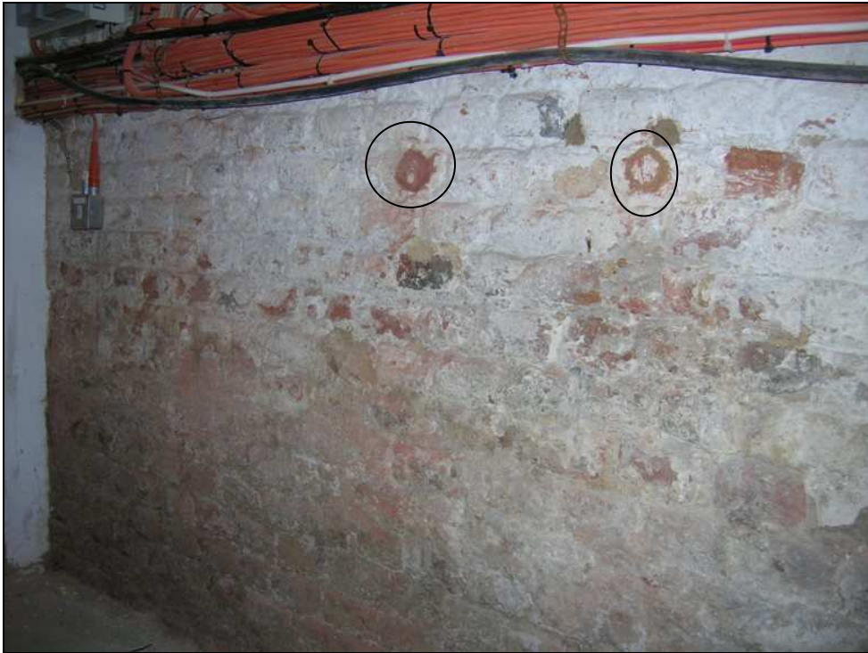
Fig. 3.19: The southern wall of the northern cellar, showing the brickwork around the sample locations. The two sample points are circled.
