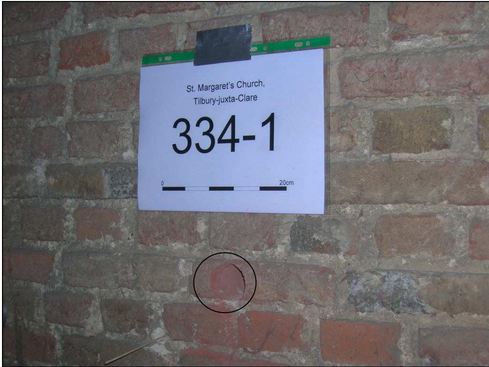
Fig. 3.117: The sample point in the western wall of the church tower. The scale is 20 cm in length. The sampling point is circled.
