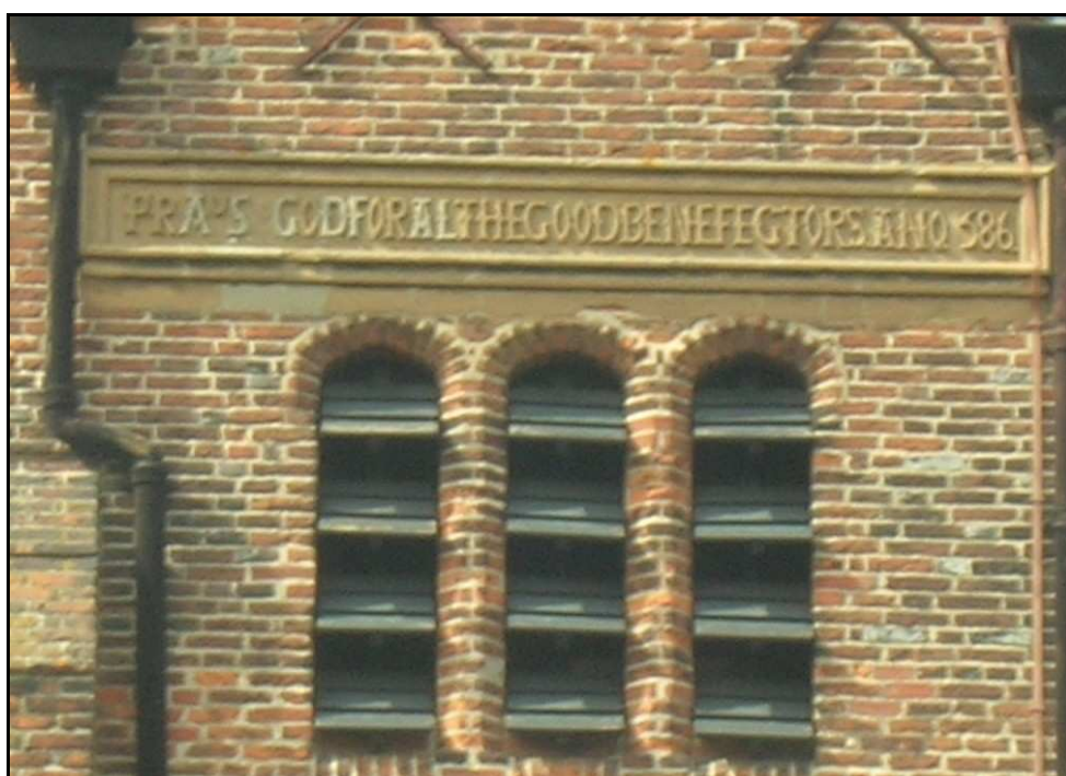
Fig. 3.99: Date plate located on the southern side of the third stage of the church tower.
