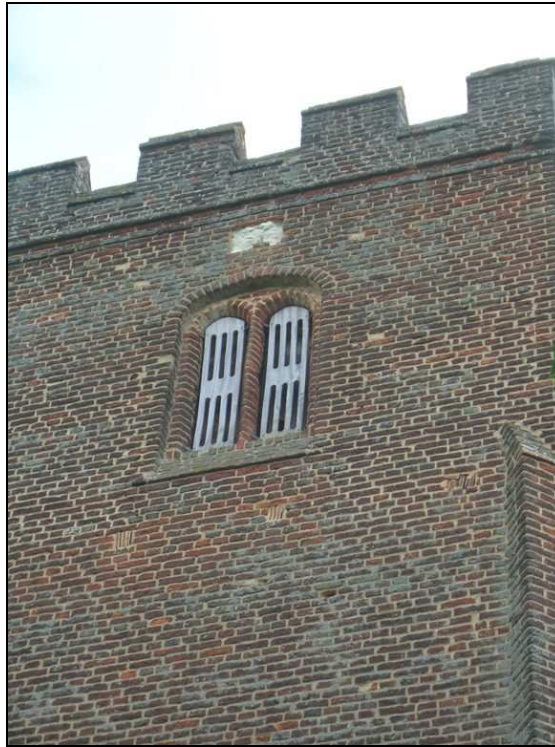
Fig. 3.114: The western face of the third stage of the tower. Note the weathered stone panel set immediately above the belfry window.
