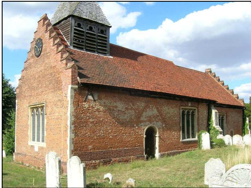
Fig. 3.119: St. Michael’s church, Woodham Walter, from the south west corner. Note the traces of plaster on the southern wall and the outline of the earlier porch roof above the southern door.
