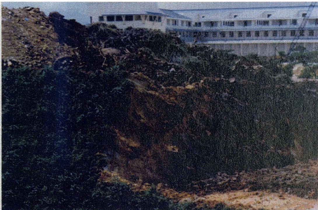
Figure 3.5 The soil profile of the NTU-CSE slope as it was revealed from nearby excavation works.
