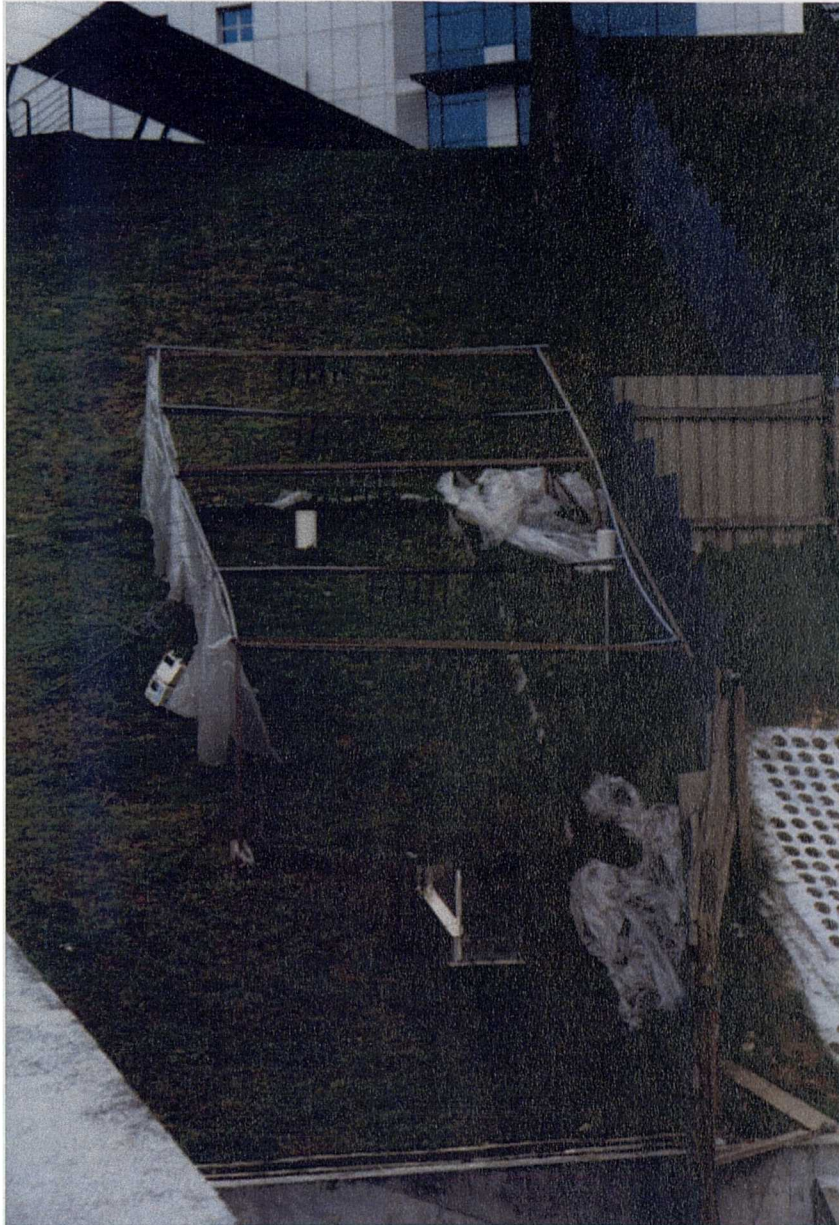
Figure 3.23 The rainfall simulator device installed on the NTU-ANX slope. Note the additional rainfall gauge installed on the research slope for measuring the intensity of the sprayed water.
