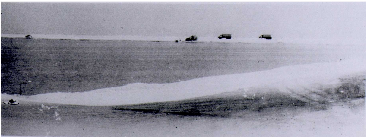
Land reclamation in progress to the seaward side of the city.
