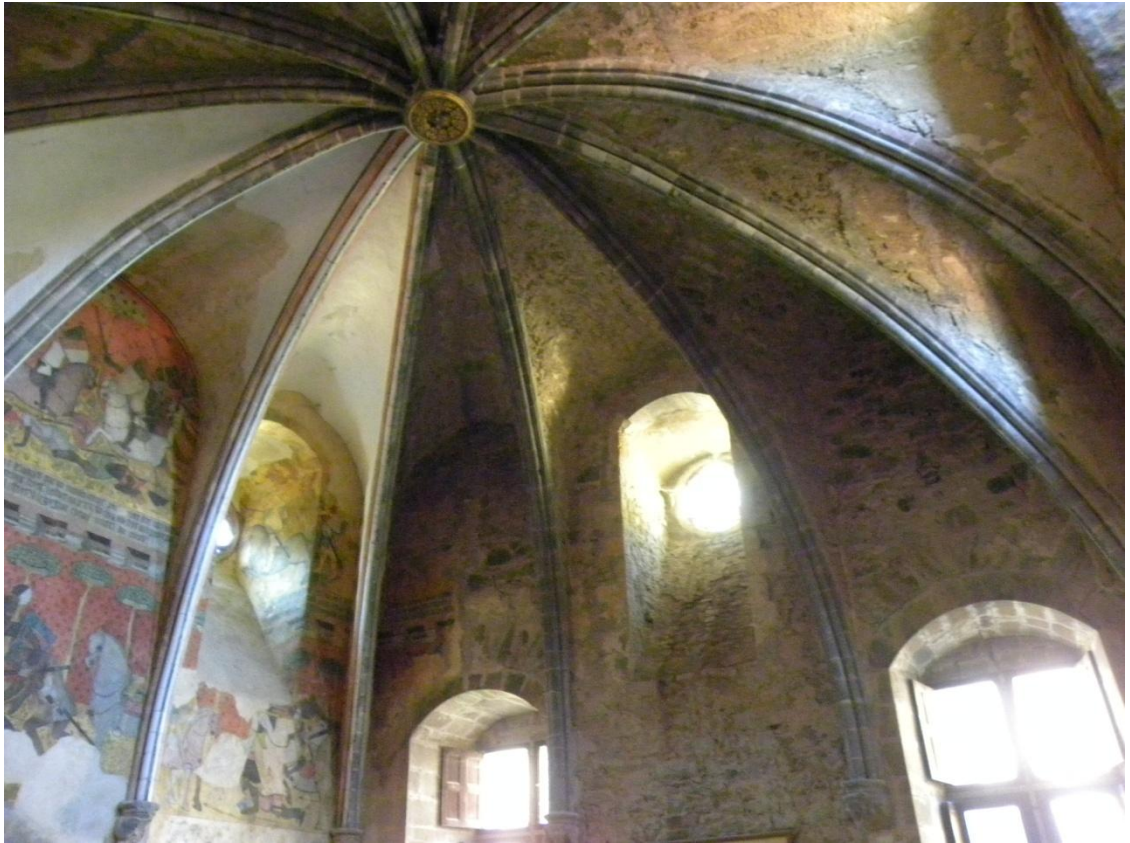
Fig. 2.23. Vaulting of main hall, with north and east walls, fresco , Château de Saint-Floret, Auvergne-Rhône-Alpes; Puy-de-Dôme, fourteenth century.
