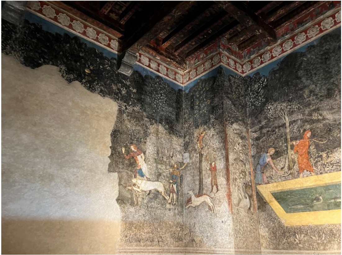
Fig. 3.33, West wall (loss where the deer would have been) and north-west corner, by Matteo Giovannetti and workshop, fresco and a secco additions, in the Chambre du Cerf, Wardrobe Tower, Palais des Papes, Avignon, c. 1343.
