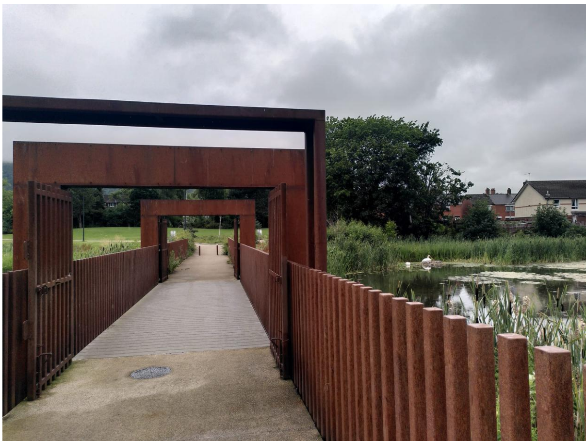
Figure 5.6: The Bridge over the Springfield Dam, and the Peace Gates which have been constructed on it. (Source: the author)
