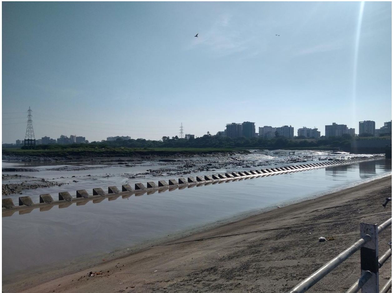
Figure 4.9: Flood embankment built after the 2006 flood
