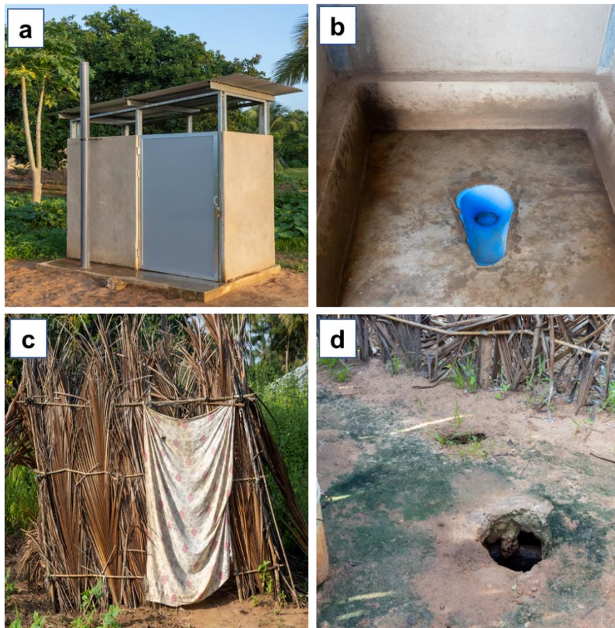
Figure 4.5: Toilet types. a) exterior of a Star home toilet, b) interior of a Star home toilet showing the main hole with a flap, c) exterior of a traditional toilet and d) interior of a traditional pit latrine showing open hole.
