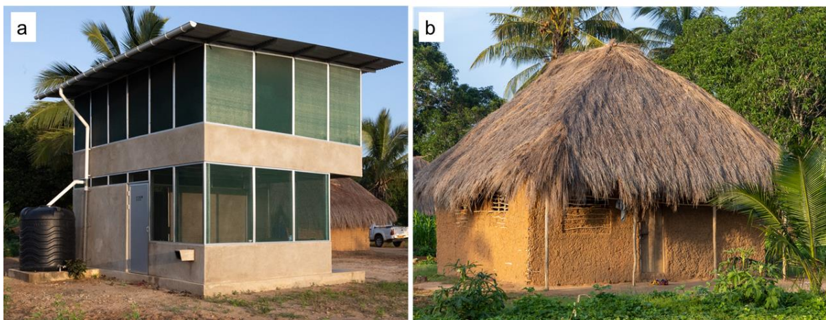
Figure 4.2: Study houses. a) Star home and b) traditional house.
