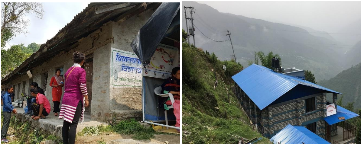
Figure 27: Picture of the old and new structure (post-earthquake) of the health centre in Sunkhani
