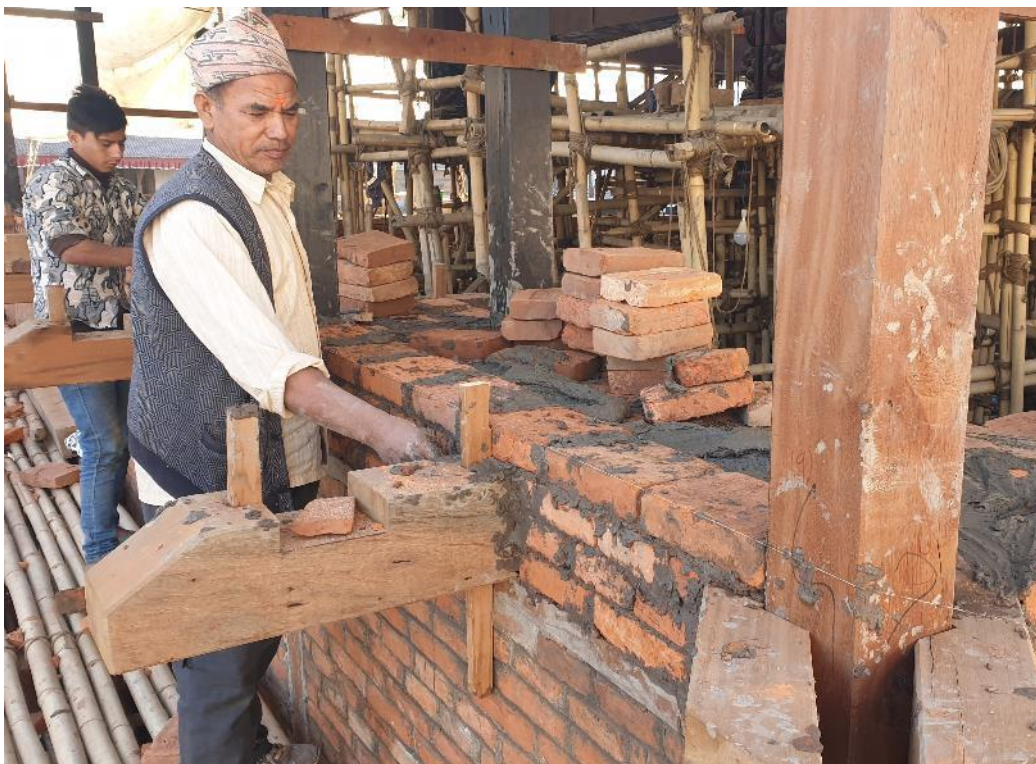
Figure 7.8: The head mason working on the brickwork integrating timber elements held in place with chukuls or pegs (Image Anie Joshi).
