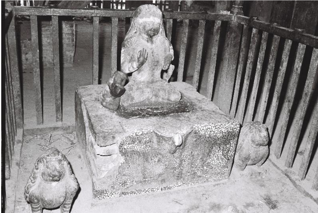
Figure 5.7: Gorakhnath shrine before the 1985 restoration (Image DOA).
