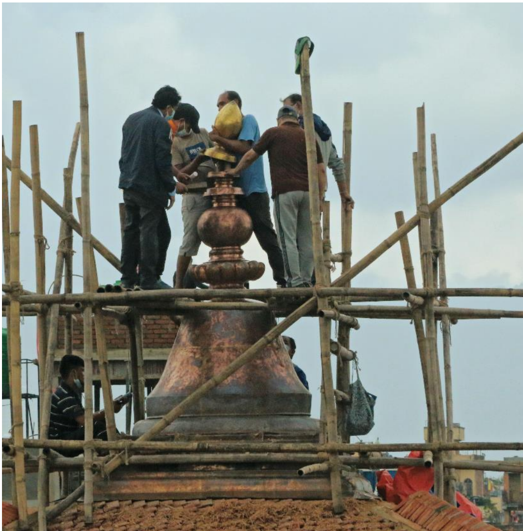
Figure 7.14: The salvaged gilded chudamani being fixed to the newly installed gajur (Image Anie Joshi).
