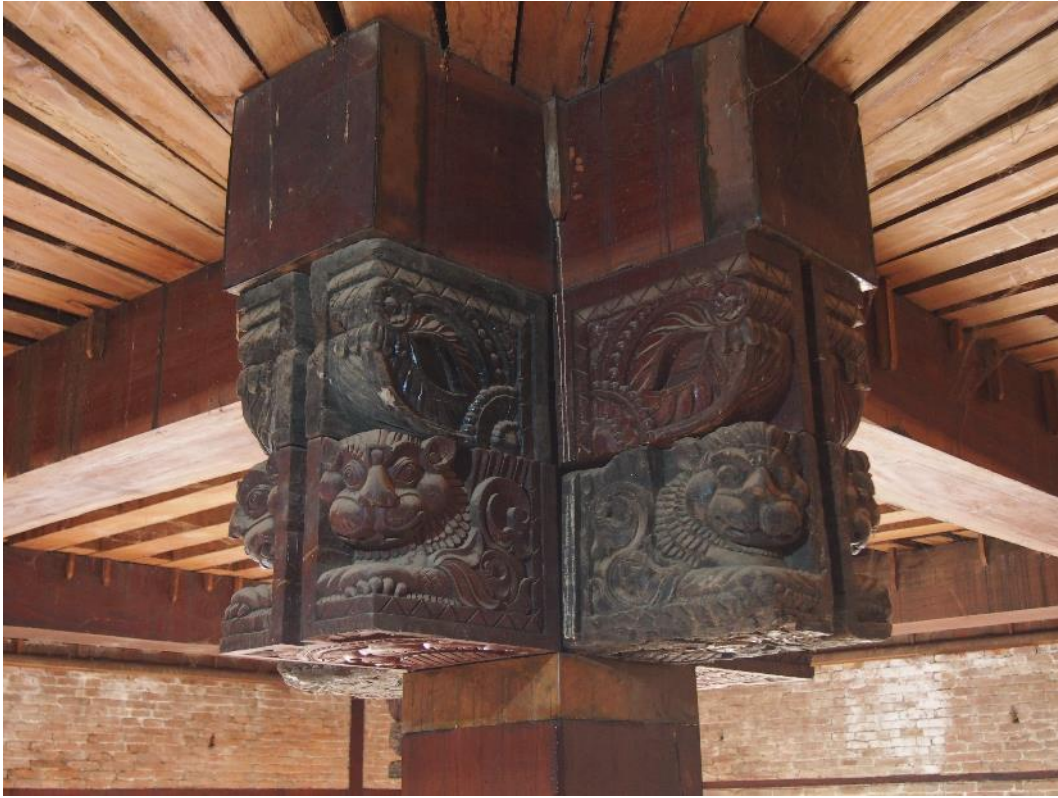
Figure 7.17: Reused fifth to sixth century CE timber bracket (Image Anie Joshi).
