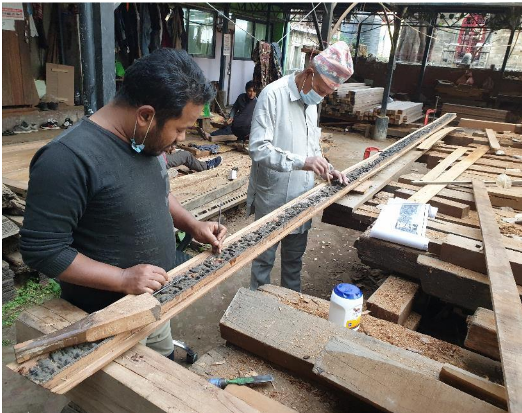
Figure 7.12: Fixing the fries connected below the pavilion balustrades (Image Anie Joshi).
