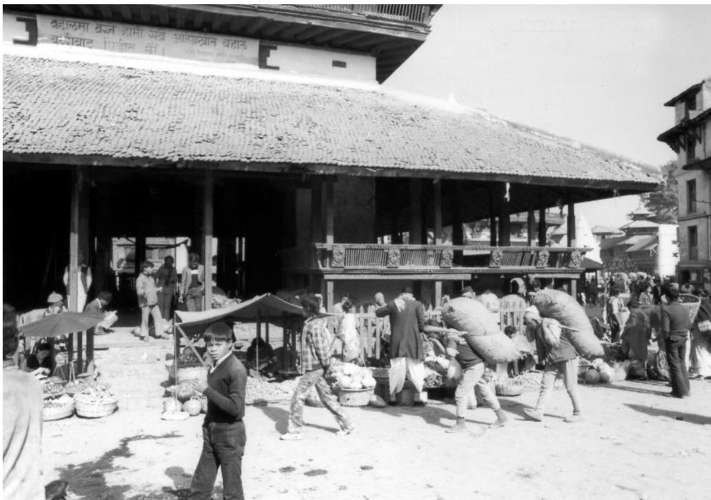
Figure 5.10: Encroachment with shop stalls and damages to the wooden elements in the early 1980s site (Image Ng Chong Kin 1983)
