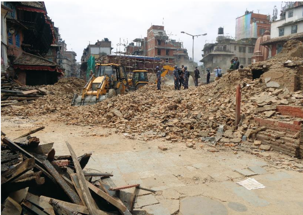
Figure 6.4: Backhoes at the Kasthamandap site on 26th April 2015 (Image Kai Weise).
