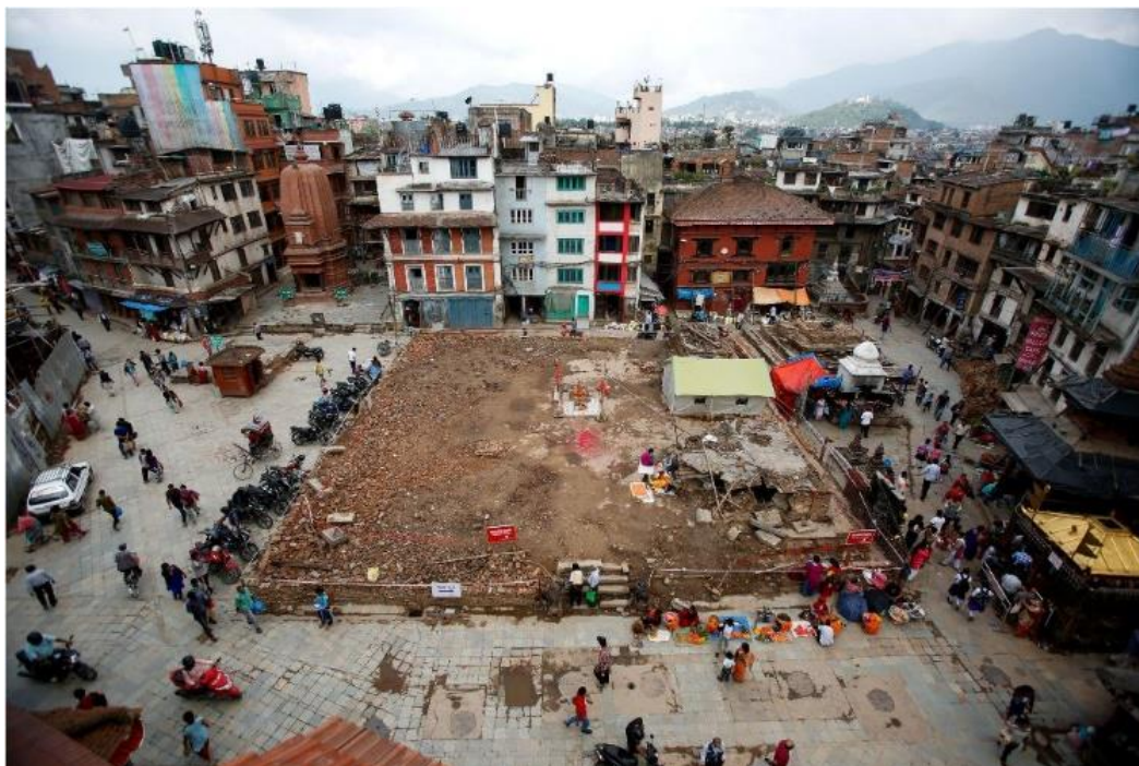
Figure 6.6: the mound of debris at the Kasthamandap is still being used by various communities (Image Kathmandu Post 30th December 2018).
