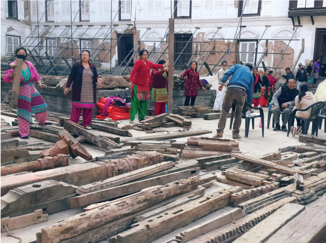
Figure 6.2: Salvaged material was stored inside the palace courtyards (Image Manindra Shrestha).
