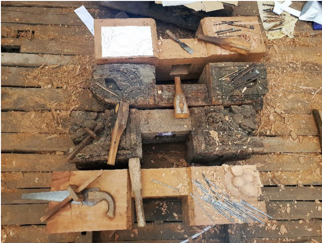
Figure 7.9: New wooden brackets being carved using old ones as templates (Image Anie Joshi).
