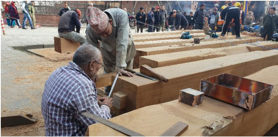
Figure 7.13: Fixing copper shoes to the main timber posts (Image Anie Joshi).
