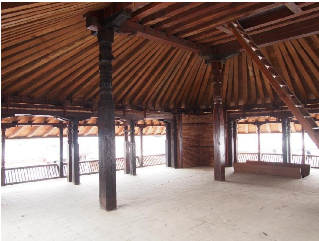
Figure 1.4: View of the upper floor of the Kasthamandap after reconstruction in 2021 (Image Kai Weise).
