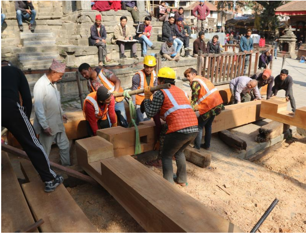
Figure 7.7: The head carpenter supervising labourers in arranging the main central beams (Image Anie Joshi).
