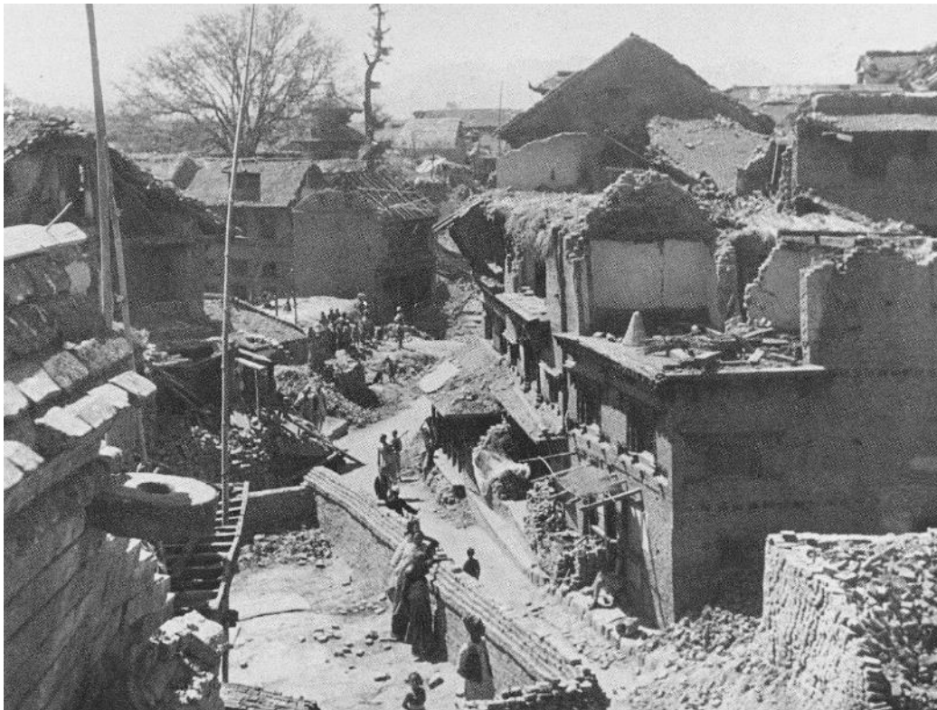
Figure 2.4: Residential areas of Bhaktapur damaged by the Great Nepal Bihar Earthquake of 1934 (Proksche 1995: 105).
