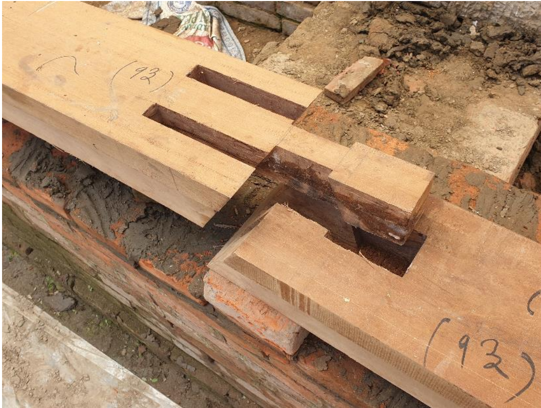
Figure 7.11: Traditional timber joint (Image Anie Joshi).
