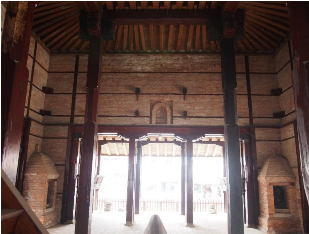
Figure 1.3: View of the ground floor of the Kasthamandap after reconstruction in 2021 (Image Kai Weise)
