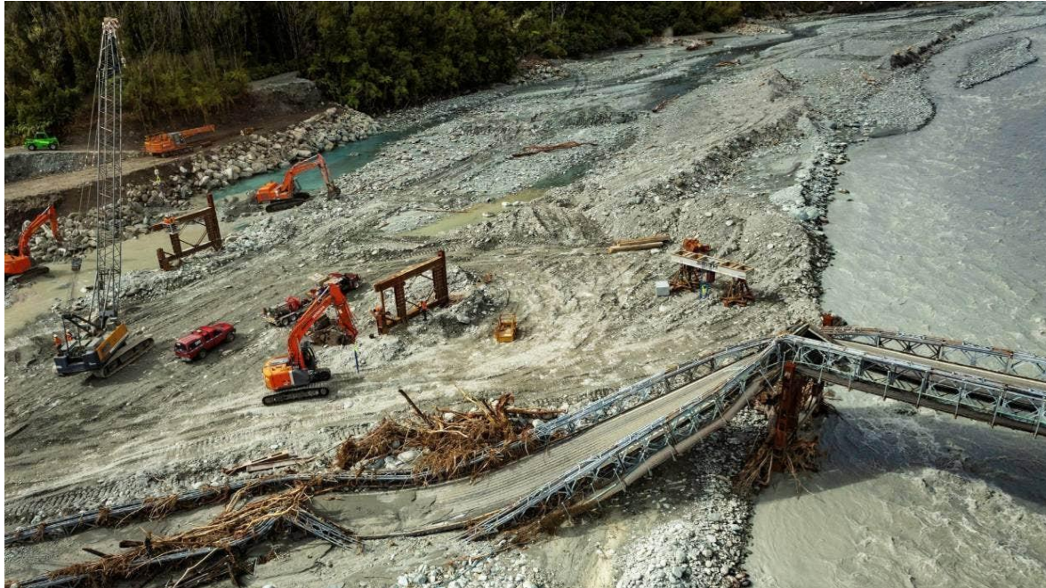
Figure 6.5. The aftermath of the flooding which wiped out the Waiho bridge (Photo credit: Stuff NZ).
