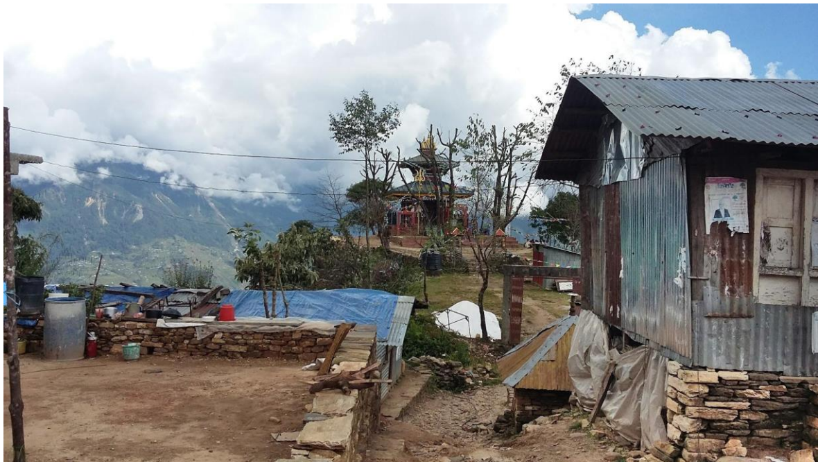
Figure 5.7. Buildings in Listi in the foreground, using brick and corrugated galvanised iron sheets and in the background, timber frames on brick (Photo credit: author, 2017).
