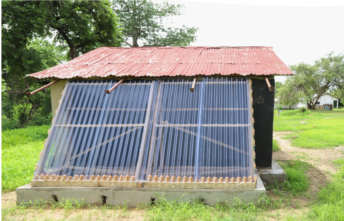
Figure 6. 3 Experimental house with solar chimney on east-facing wall.
