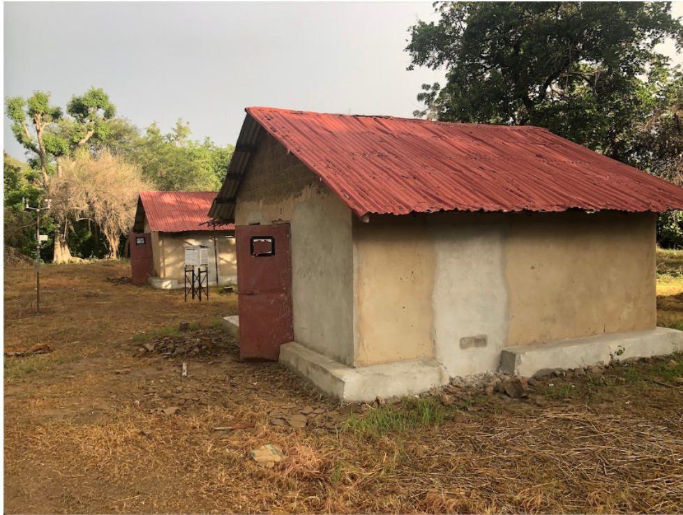
Figure 5. 3 Experimental houses with one door and one window on the front and rear facades.
