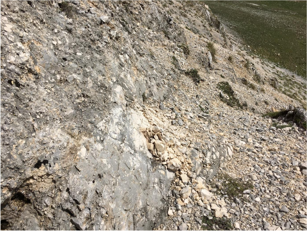
Footwall bedrock with eroded sections, looking SE
