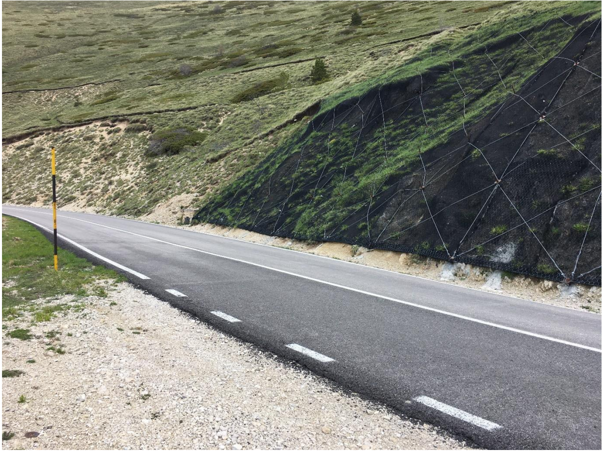
Resurfaced road and hillside protection, looking W
