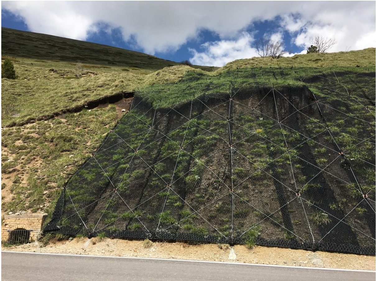
Hillside protection, looking N
