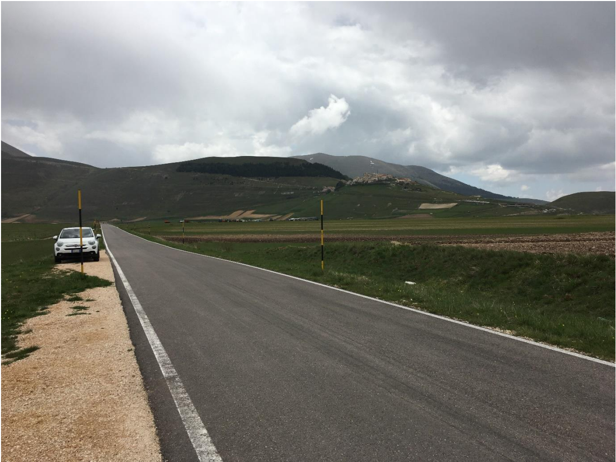
Resurfaced road, looking W
