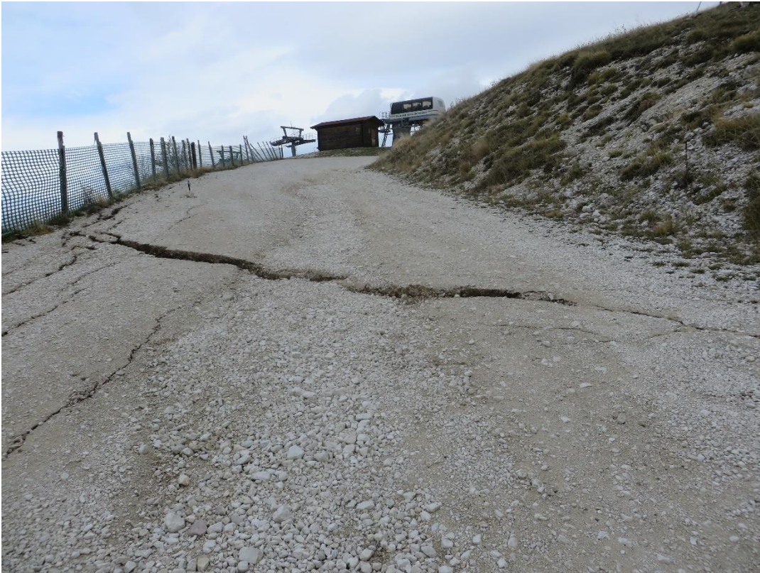
Figure 124: Rupture from Norcia earthquake across gravel access track looking north to Bove Rd ski lift, taken on 5 th November 2016 at ~UTM 33T 351007/4752687 (photograph by Luke Wedmore, then University of Leeds, now University of Bristol).
