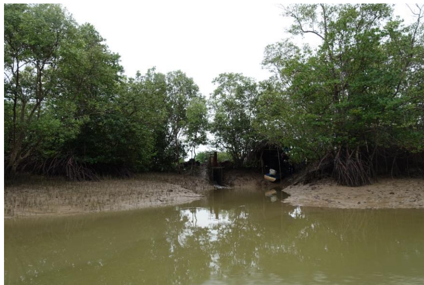
Figure 41 A sluice gate from the view of the river during the low tide
