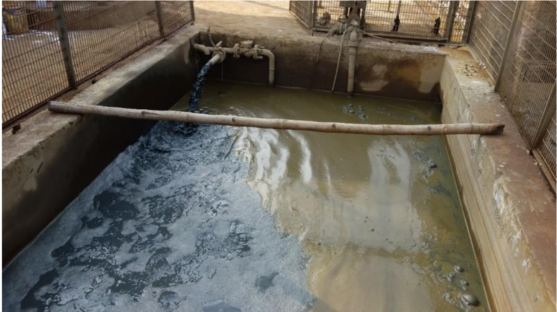
Figure 1: Wastewater basin at a small factory in rural India; photo taken in February 2020. The water contains high chromium concentrations and is only treated rudimentarily before being released into the environment.
