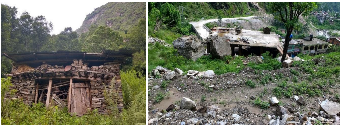
Figure 5-15. Impact of the earthquake-induced landslides and resultant direct rock falls on a person's house.
