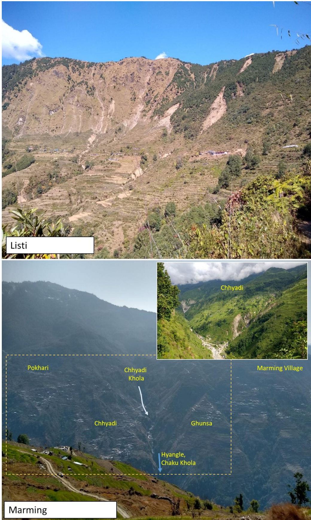
Figure 3-9. Glimpse of two off-road communities located on the mid-slope of a hill in the Upper Bhote Koshi Valley.
