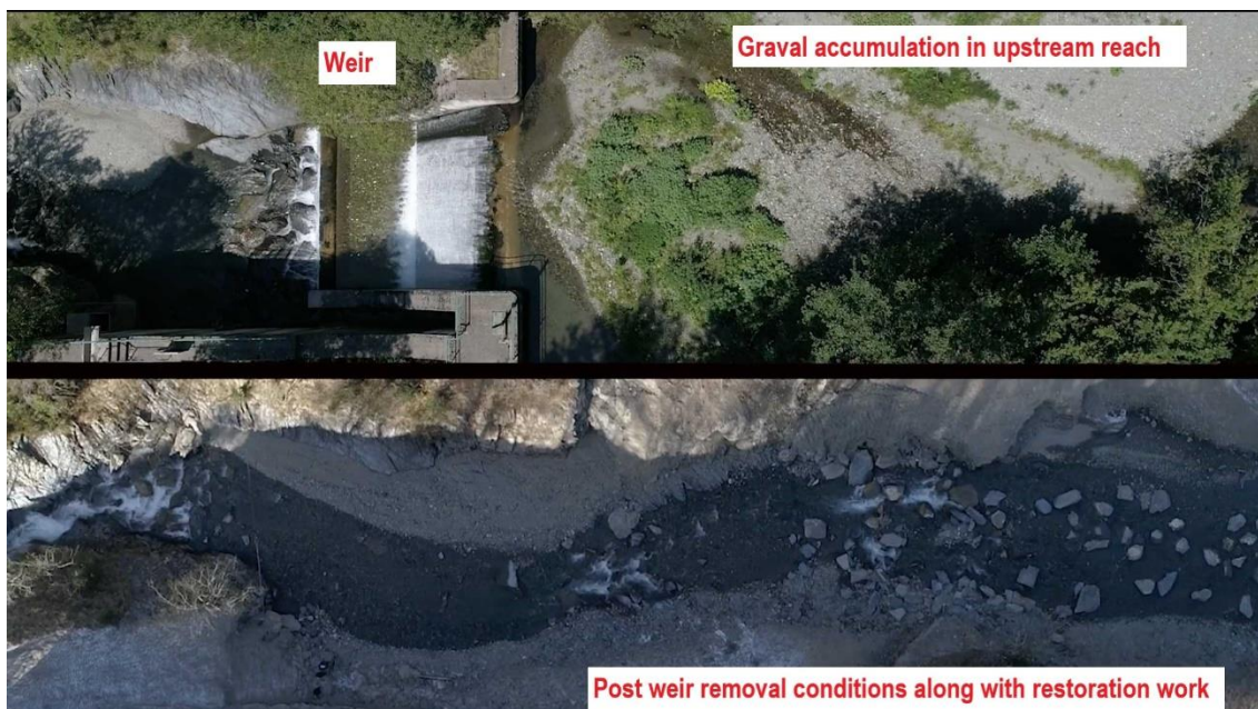
Figure 1.7 Weir removal (also known as Mollo Dam) at the Ritort River (Spain) shows upstream gravel accumulation and local base-level changes while the weir was functional.
