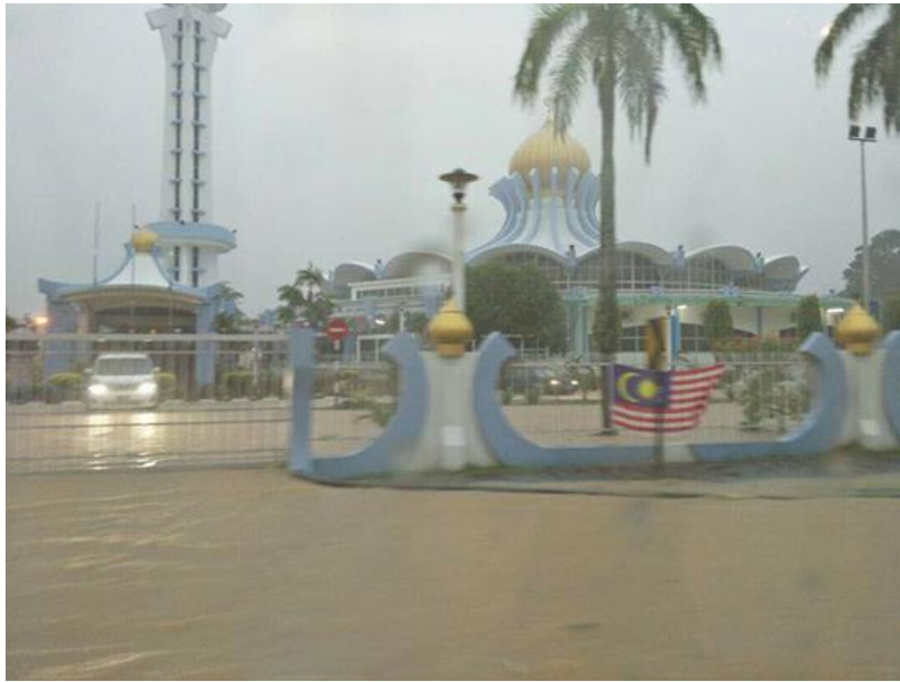
Figure 6.6: Heavy rainfall blocked the drainage system in Penang
