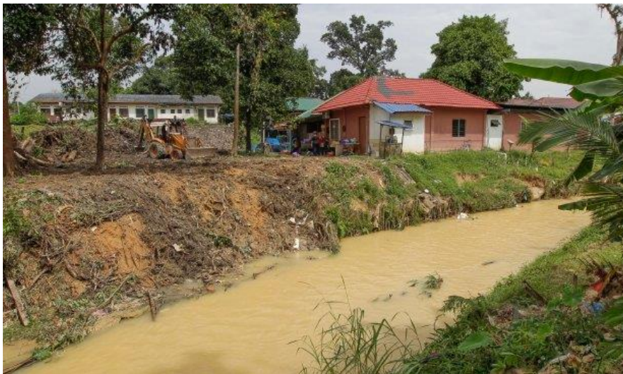
Figure 6.7: One of the mitigation projects in Nelayan Village, Teluk Kumbar
