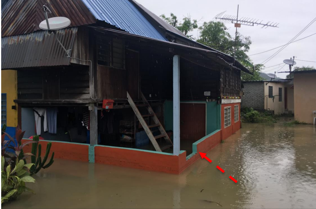
Figure 5.3: House built with retention wall at surrounding
