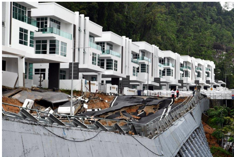
Figure 6.5: Existing and new property and infrastructure destruction caused by flood
