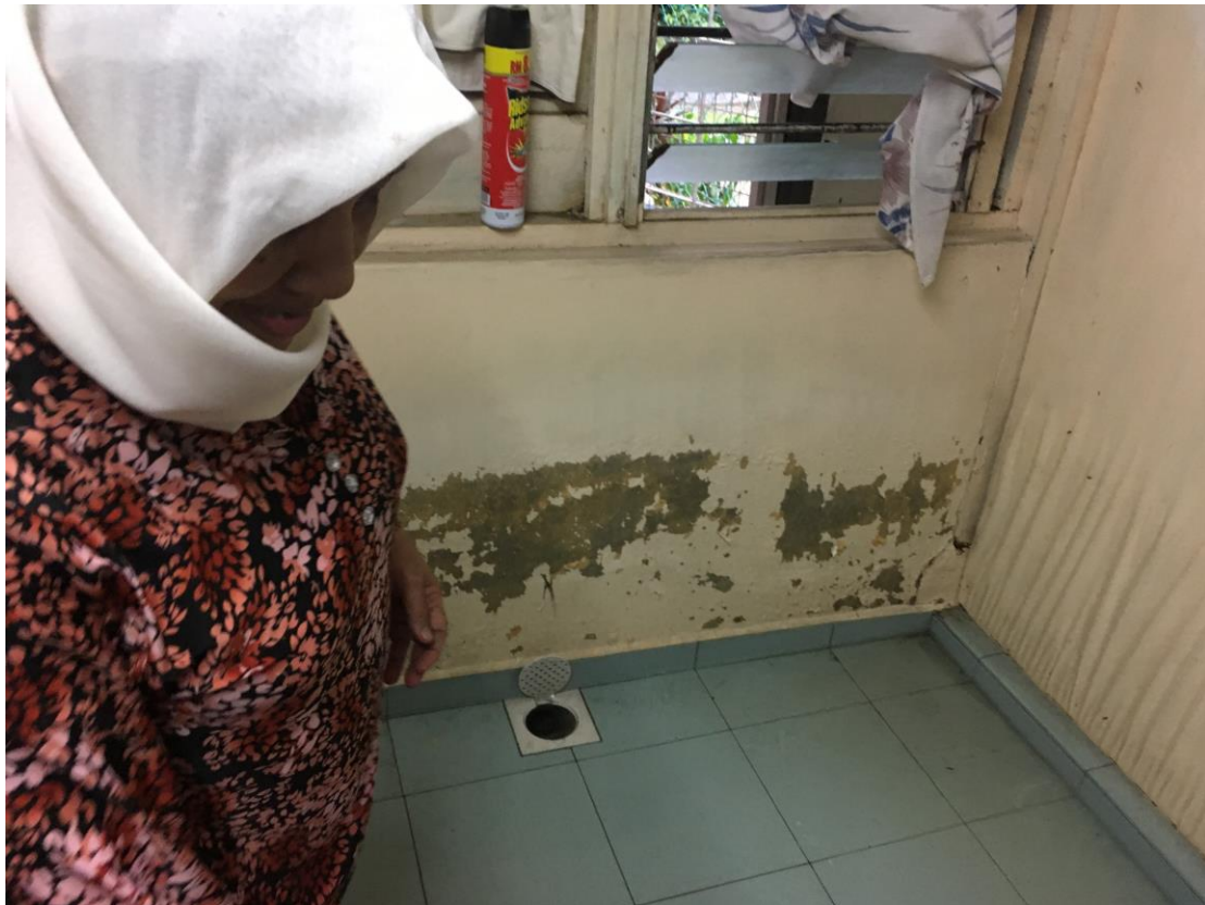
Figure 5.1: Resident showing one of their coping - water drain idea
