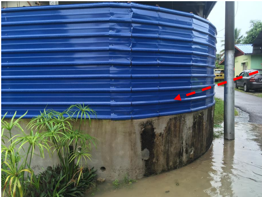
Figure 5.4: Houses in Teluk Kumbar with retention wall and raised high platform
