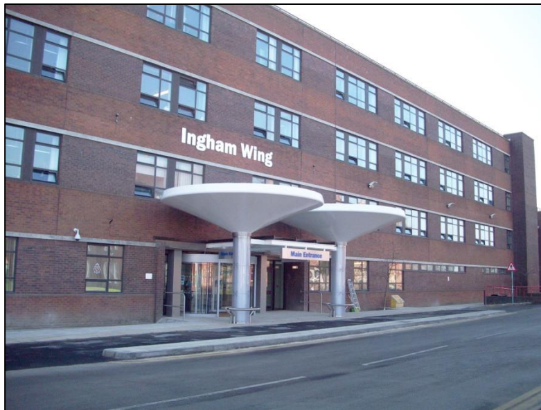
Figure 6.1: South Tyneside District Hospital (Ingham Wing).
