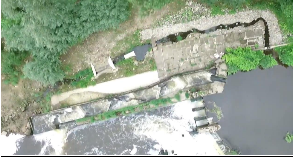
Figure 2.5: Birds eye view of the Salmon ladder and semi-formalised nature-like bypass at Naburn. Reproduced from ( www.youtube.com ).
