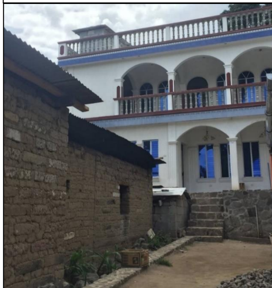
Figure 55: Contrasting traditional and modern architecture
