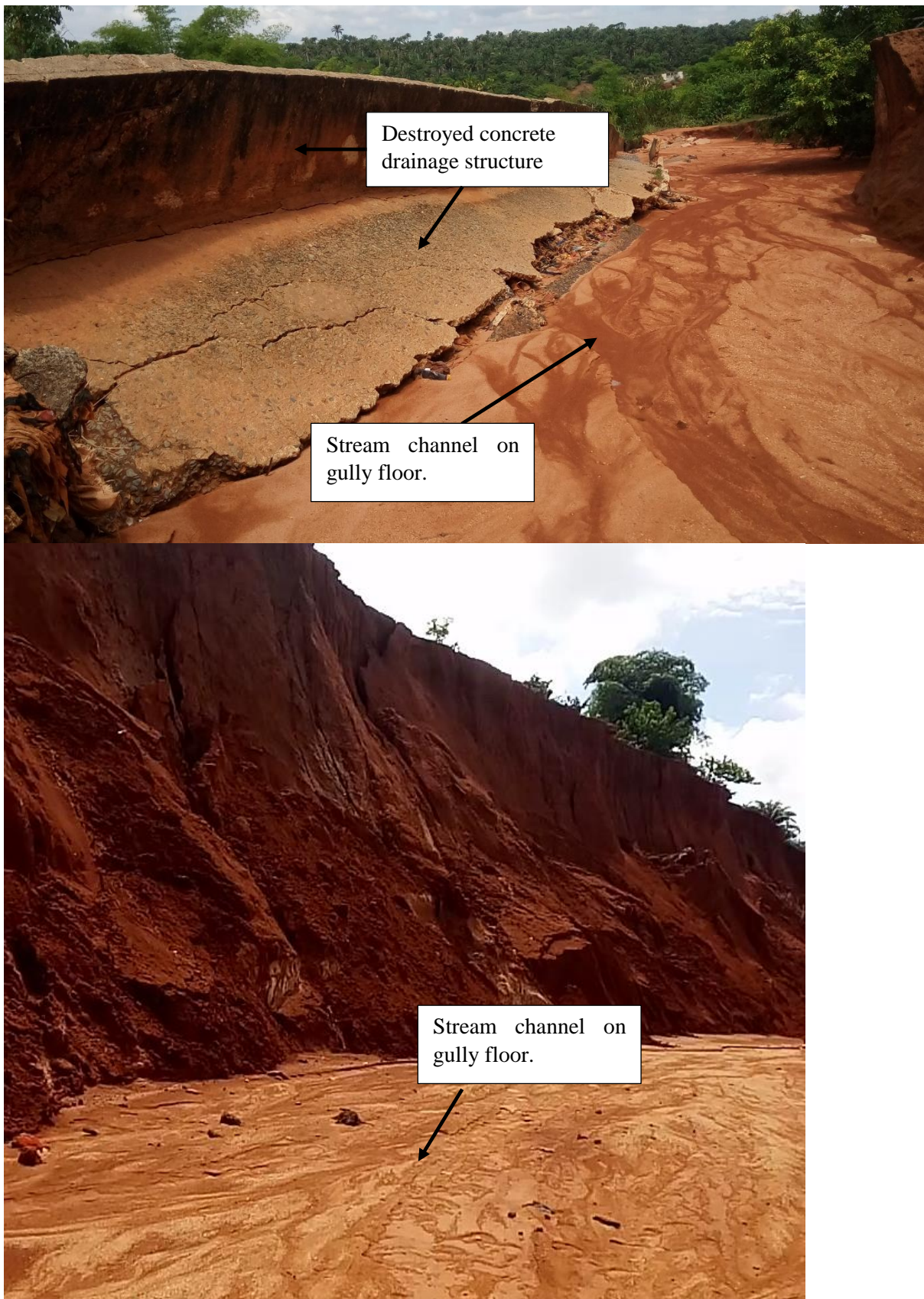
Figure 6.13: Evidence of streamflow on gully floors at the younger Obibi-Ochasi gully. Also shown is a destroyed drainage structure designed to transport runoff to a local base level.
