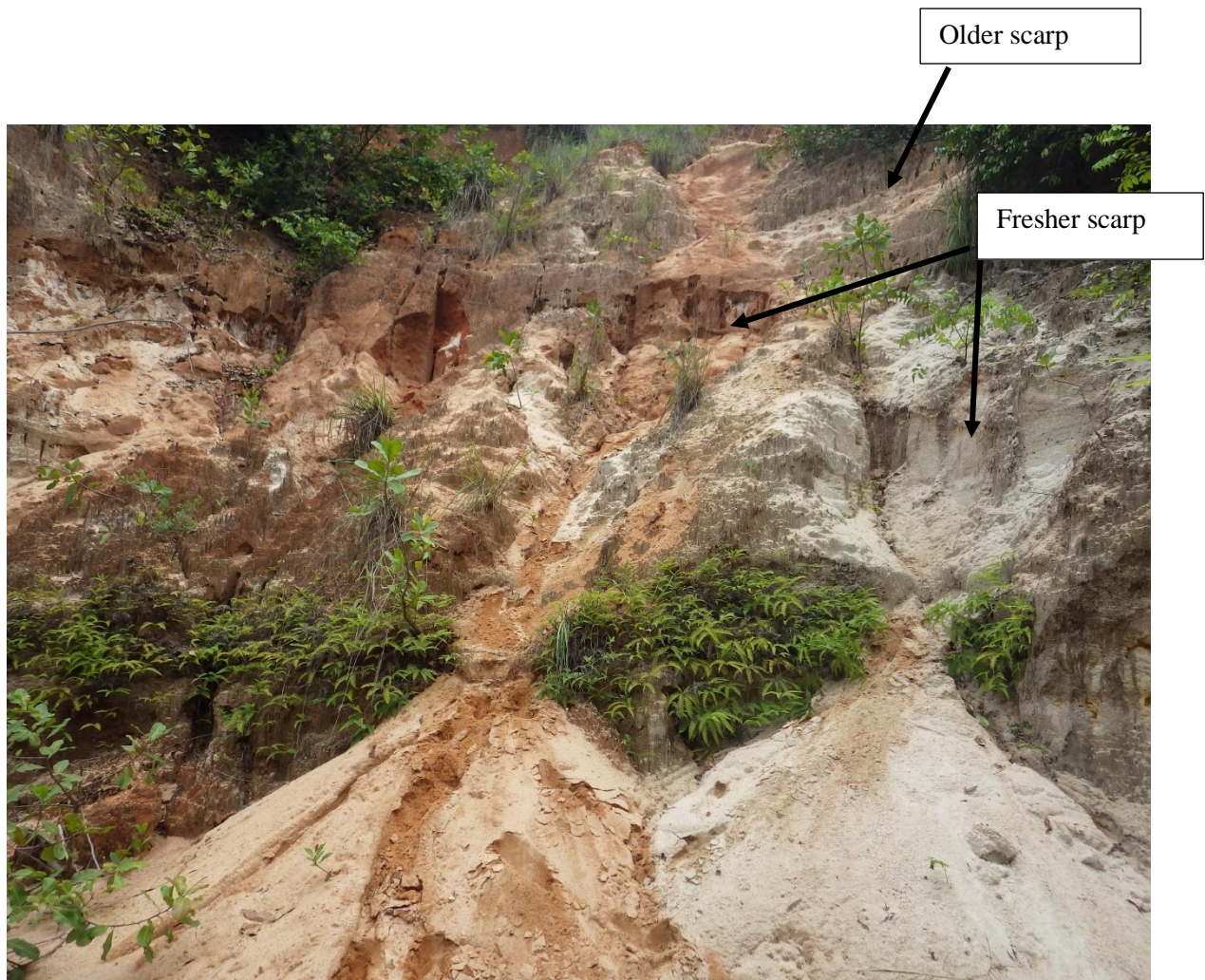
Figure 6.2: Gully-induced slide showing multiple failures within the Amucha gully (slide 1 of Table 6.2), location: 05.73569N, 007.03989E.
