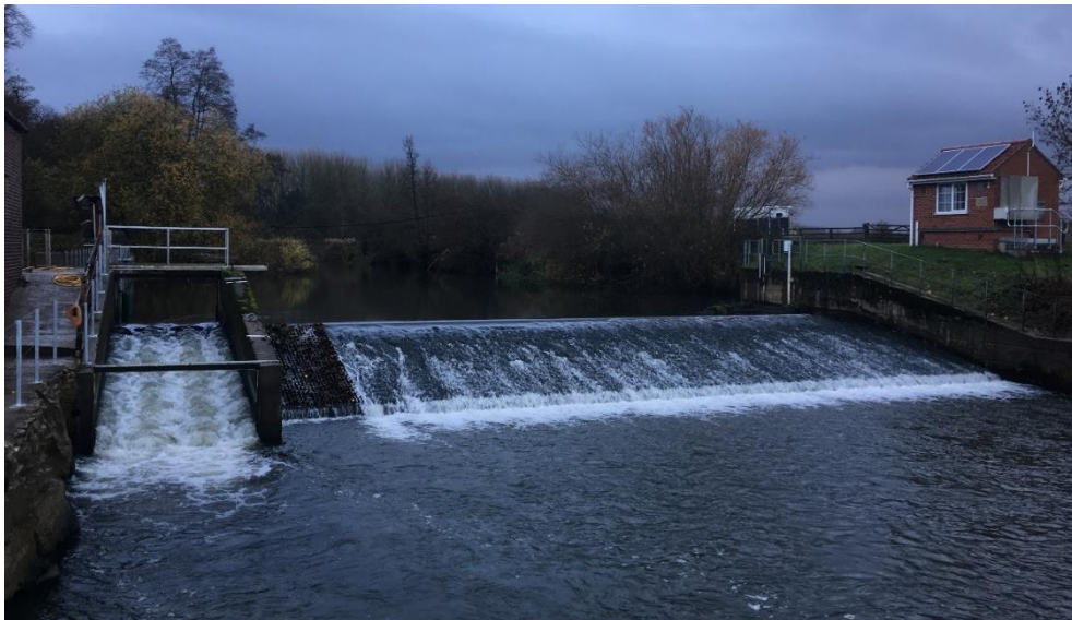
Figure 2.16. Top: Photograph of Buttercrambe gauging weir with turbine house, turbine tailrace, Larinier fishway, and horizontally-mounted tile (Photo Credit: Angus J Lothian). Bottom: Photograph of Buttercrambe gauging weir with exposed truncation of the downstream weir edge (Photo Credit: Angus J Lothian).
