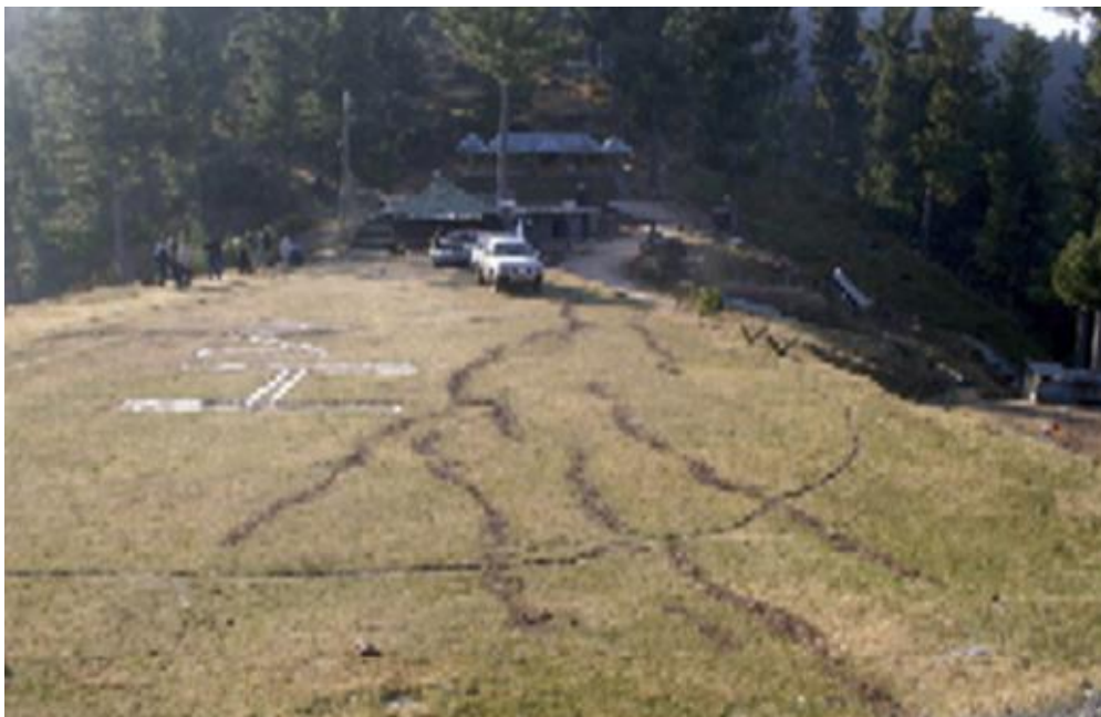
Fig. 2.13: Fissuring resulting from the 2005 Kashmir Earthquake, Pakistan. Full credit to Owen et al. (2008) – reference in bibliography. Digital enhancement of the image has been tried, but to no avail as this is the quality at which they were initially published.
