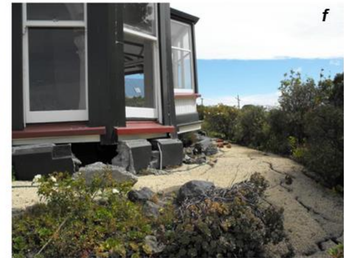
Figs. 3.08a-f: Examples of ground cracking in Christchurch which manifested during the Canterbury Earthquake Sequence in 2010-11. Documented by Dellow et al. (2011). Full credit to Dellow et al. (2011) – reference in bibliography.
