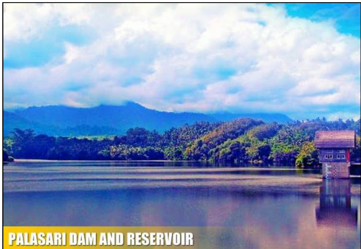
Figure 3.2 Palasari dam and reservoir
