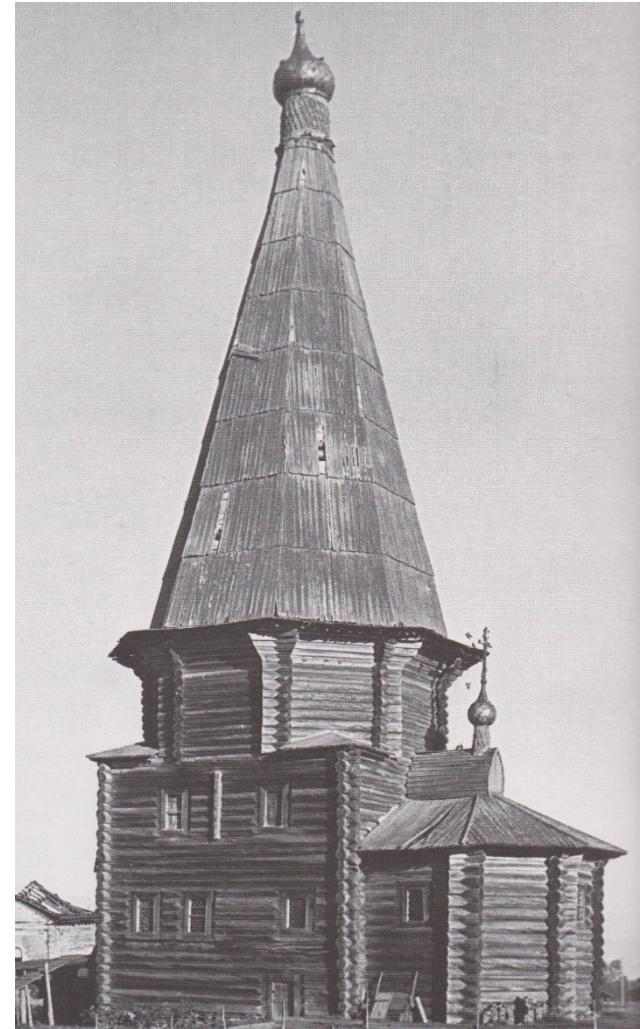
This is the form at its most basic. The square structure can be seen under the octagonal tower. The pyramidal roof and its flat sections can be clearly seen. This is St Demetrius of Salonica, Verkhnyaya Uftyuga, Russia . Photo source: Brumfield 2004: 194.
