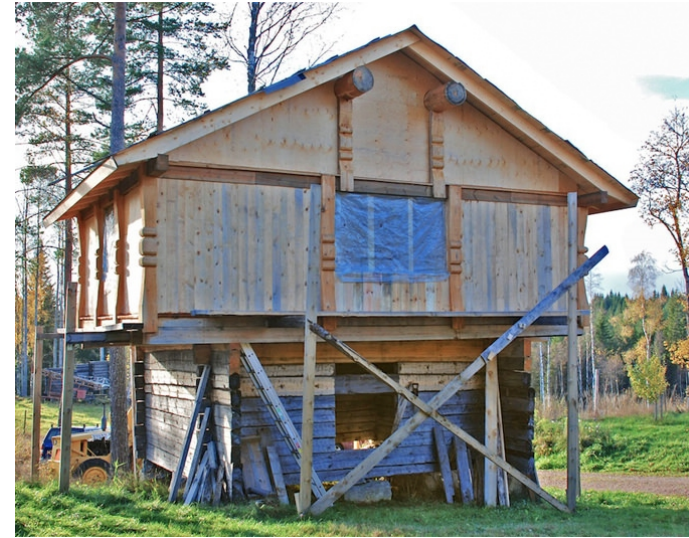
Modern loft under construction (2017). Source: www.joystudiodesign.com/norwegian/norwegian-loft-ladder.html [Accessed 06 June 2017].
