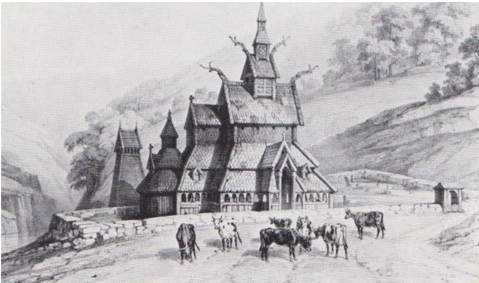
Borgund Stave church c. 1839. Drawing by A. Mayer, for P Gaimars Voyage en Scandinavie (1839: 40,41), secondary source: Christie 1978: 47.
