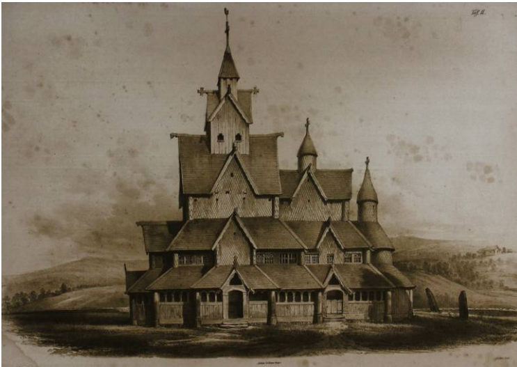
Heddal Stave Church in 1837. Source: Dahl 1837: Plate2.
