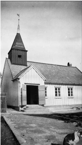
Grip Stave Church in 1923. This is before the 1930's renovations that were done to reverse the earlier renovations from the 1870's. Externally this can be seen in the different turret structure and the windows. From the personal photo collection of Kristian Berge, source: < https://www.flickr.com/photos/fylkesarkiv/8422944209/in/photostream/ > [Accessed 25 January 2015]
