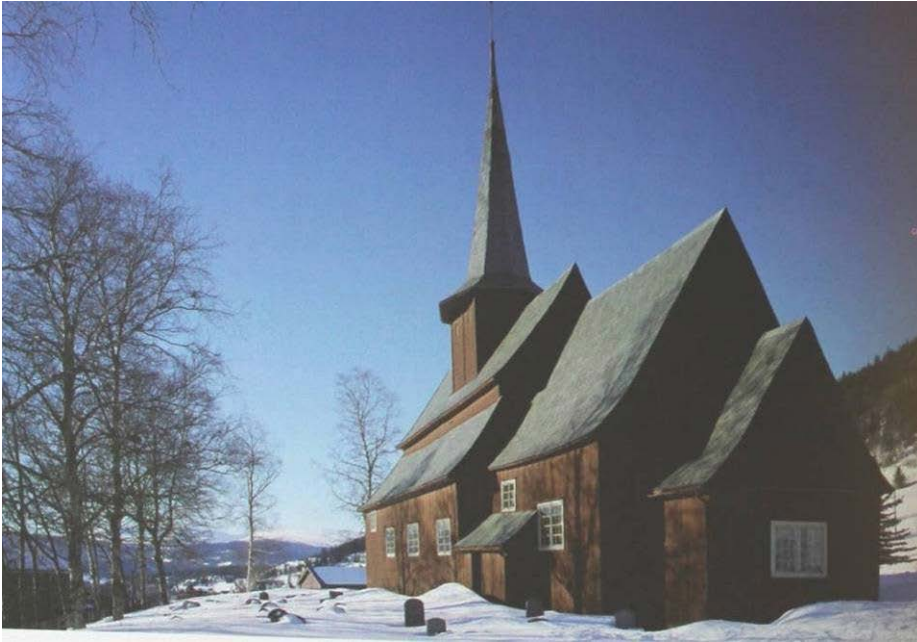
Hegge Stave Church. Source: Anker and Havran 2005: 250.
