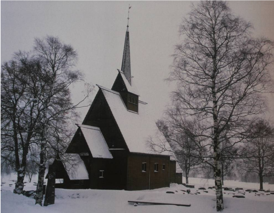
Høyjord Stave Church. Source: Anker and Havran 2005: 210.
