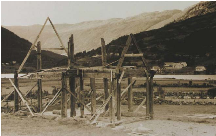
Øye Stave Church in 1960 with the original 156 discovered parts reconstructed. Used with permission from the Directorate for Cultural Heritage.
