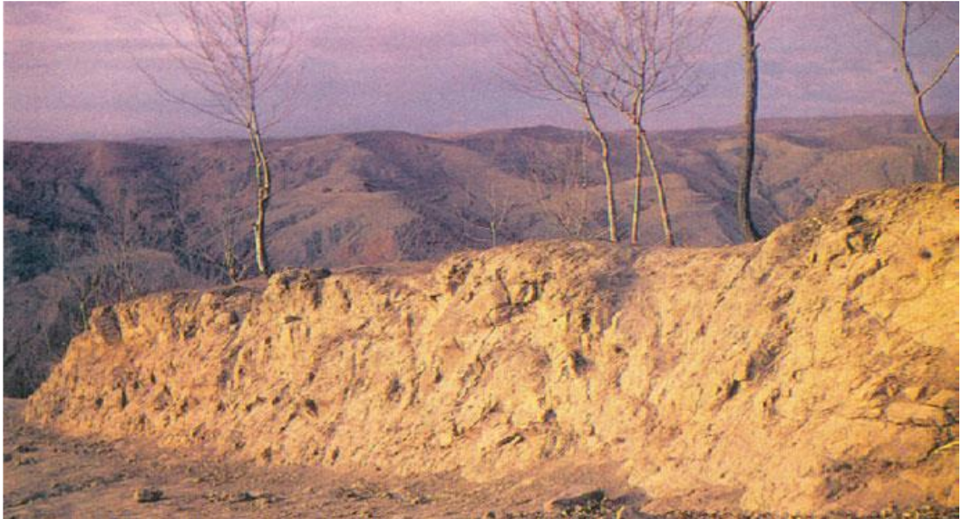
Figure 1.5: Section of the Great Wall of China built using the rammed earth technique around 2000 years ago (from Schroeder, 2016).
