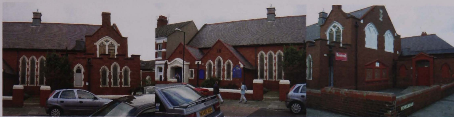
Figure 1.14 Photographs of Sandyshore Christian Fellowships' building, Sandyshore
